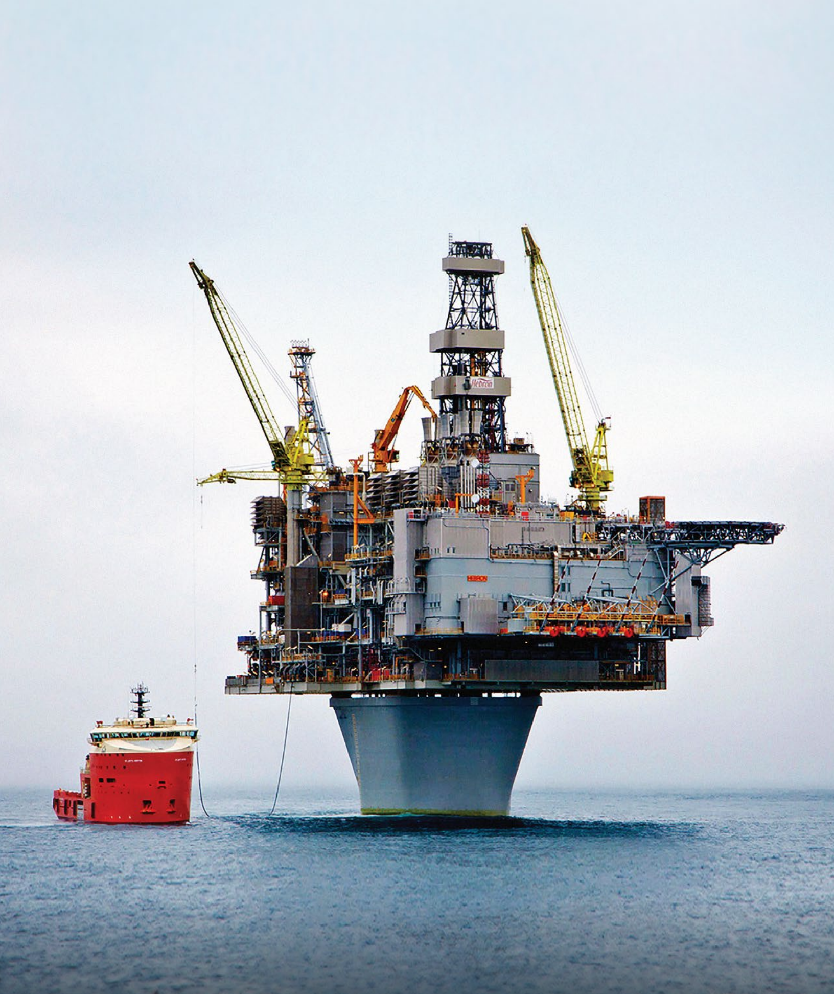
Hebron platform located offshore Newfoundland and Labrador Credit: ExxonMobil Canada
