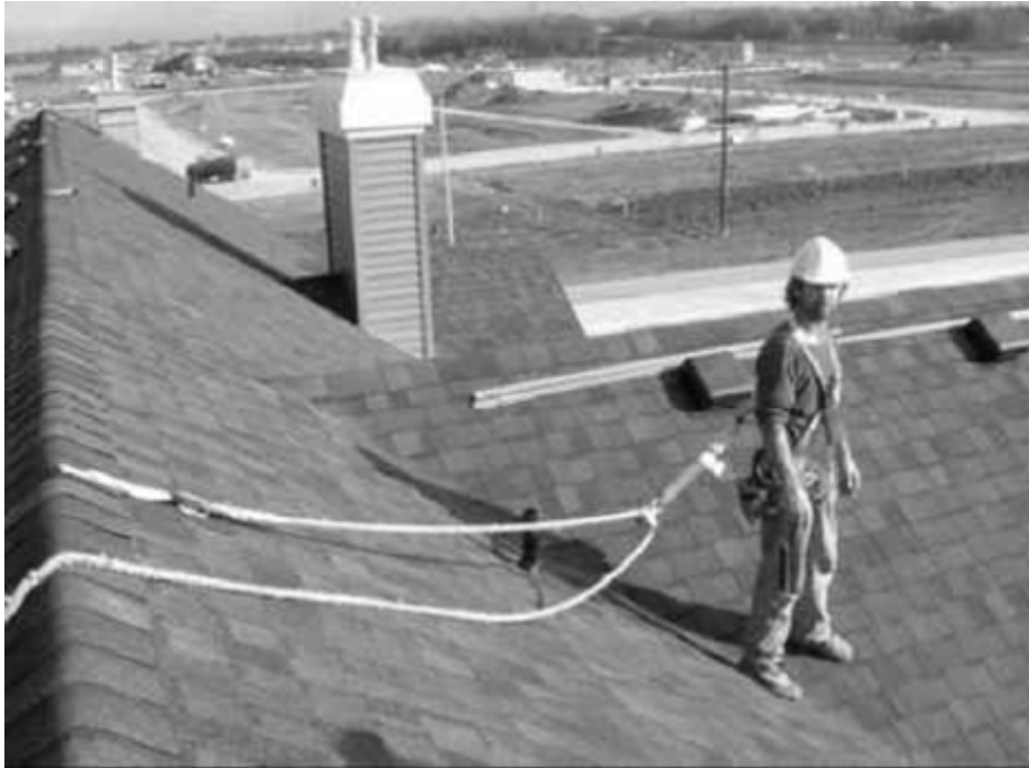
Figure 10.5 Another example of a Fall Arrest System
