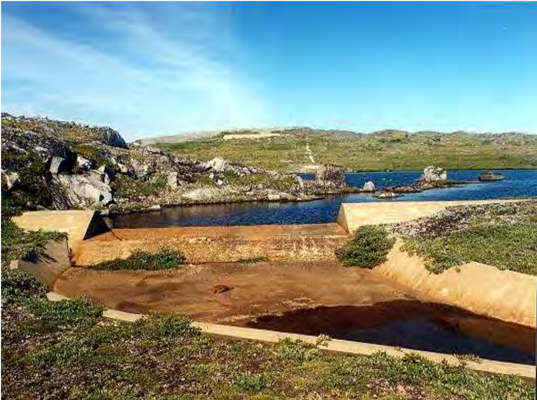
Photo 9: View, looking north, toward the dam/spillway – August 2000.
