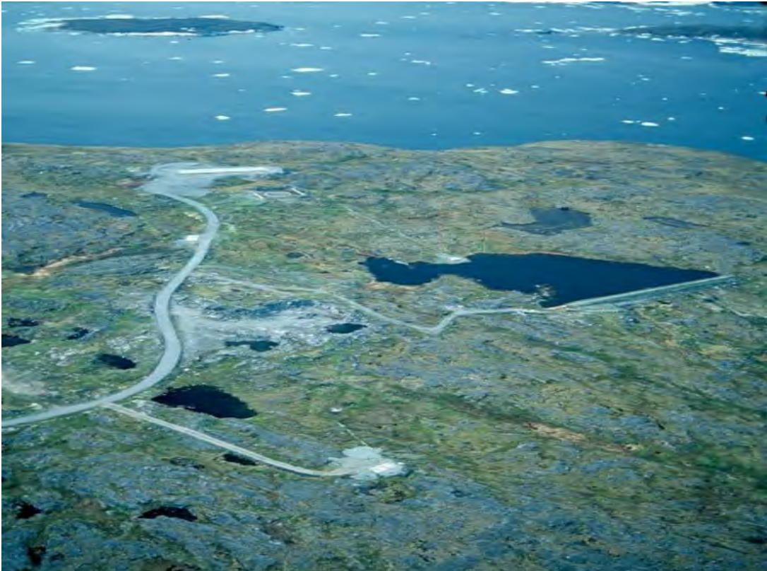
Photo 11: View, looking north towards the Site following the decommissioning activities – July 2002
