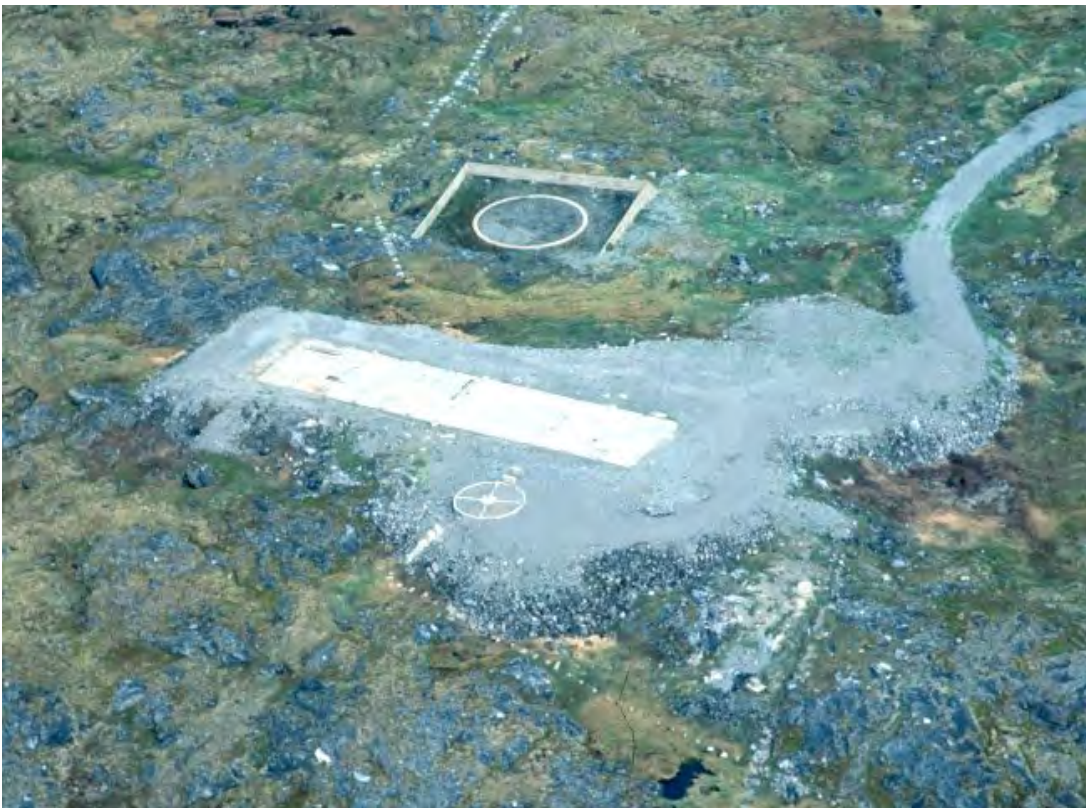
Photo 12: View, looking east, toward the remains of the radar tower, the main building and the POL fuel tank area – July 2002
