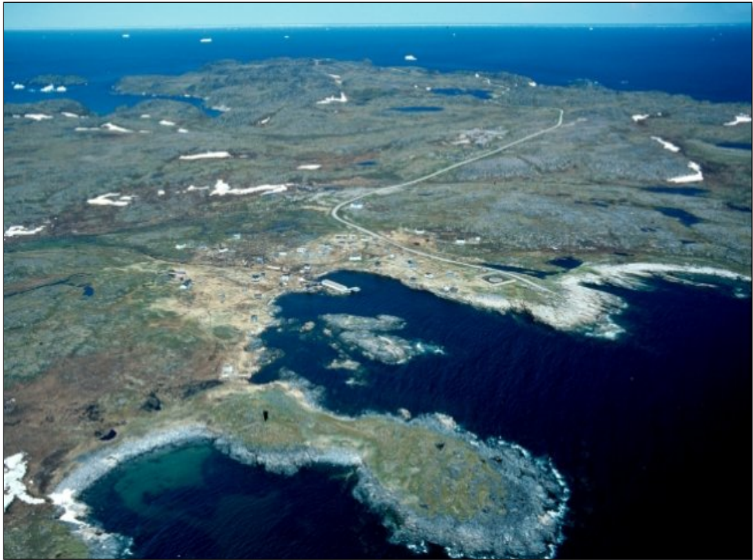
Photo 7: View, looking north, towards the village of Spotted Island. Note the gravel road from leading from the lower POL to the upper portion of the Site – July 2002.
