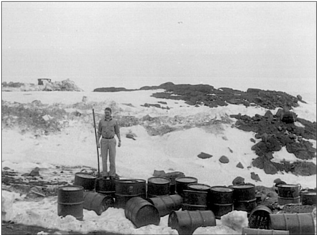
Photo 6: View, looking northeast, towards the Diesel Operator standing on the POL drums – October 1958.
