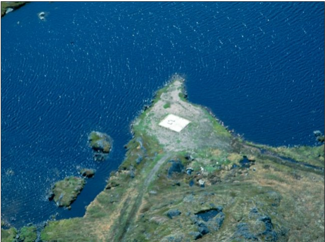
Photo 12: View, looking south, toward the remains of the former lower POL aboveground storage tank area – July 2002.
