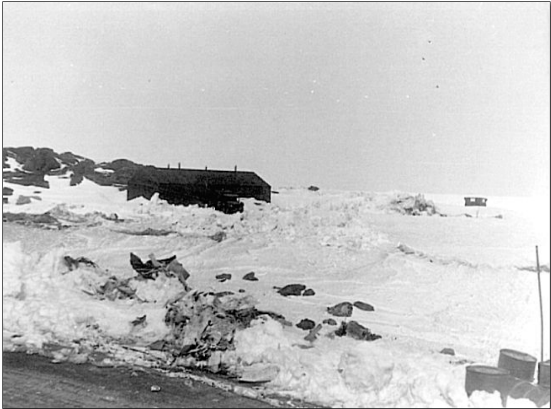
Photo 5: View, looking west, towards the disaster shack which housed an emergency generator, a radio, rations and arctic survival gear. Note the POL drums stored along the roadside in the foreground of the photograph – October 1958.
