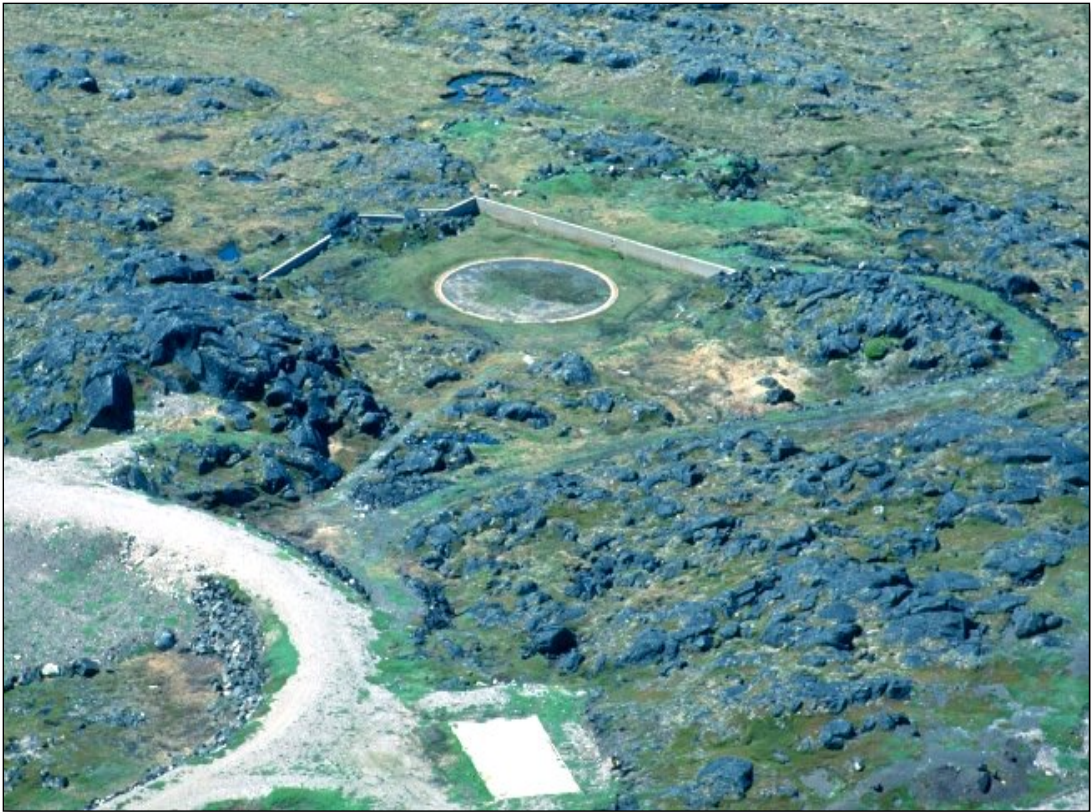
Photo 11: View, looking west towards the former upper POL aboveground storage tank area. Note the concrete foundation of the former disaster building in the foreground of the photograph – July 2002.
