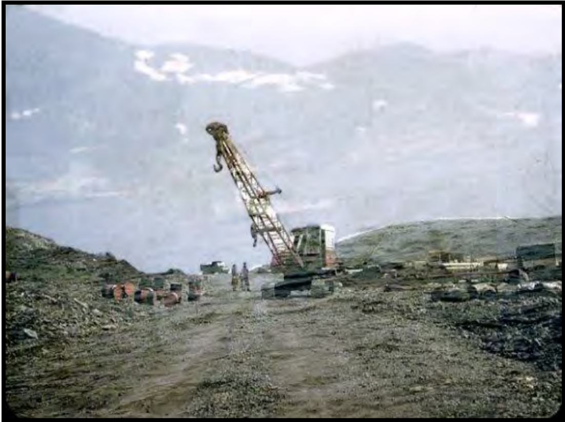
Photo 1: View, looking east, towards the steam shovel used during road construction on the hill near the site circa 1955. Note the POL drums scattered along the roadway.
