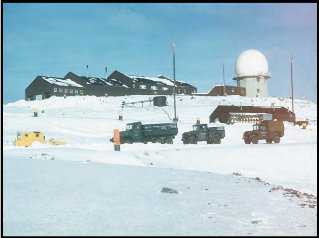
Photo 11: View, looking northwest, towards the Site from the helicopter pad - February 1960. Note the large amount of POL drums located adjacent to the disaster shack in the background of the photograph.
