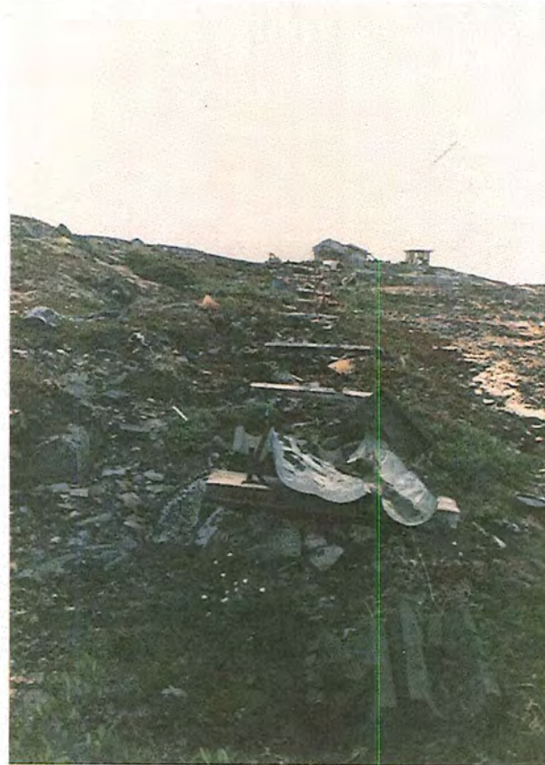
Photo #5: Water Pipeline "Aillik"
