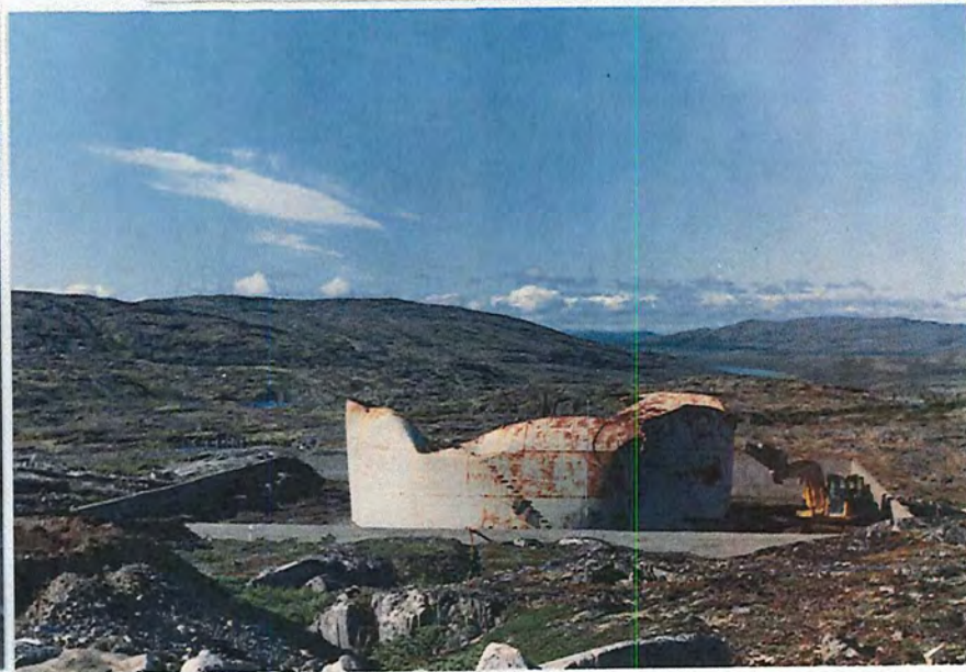
Photo #2: Cleaver Dismantling Tank "Aillik"
