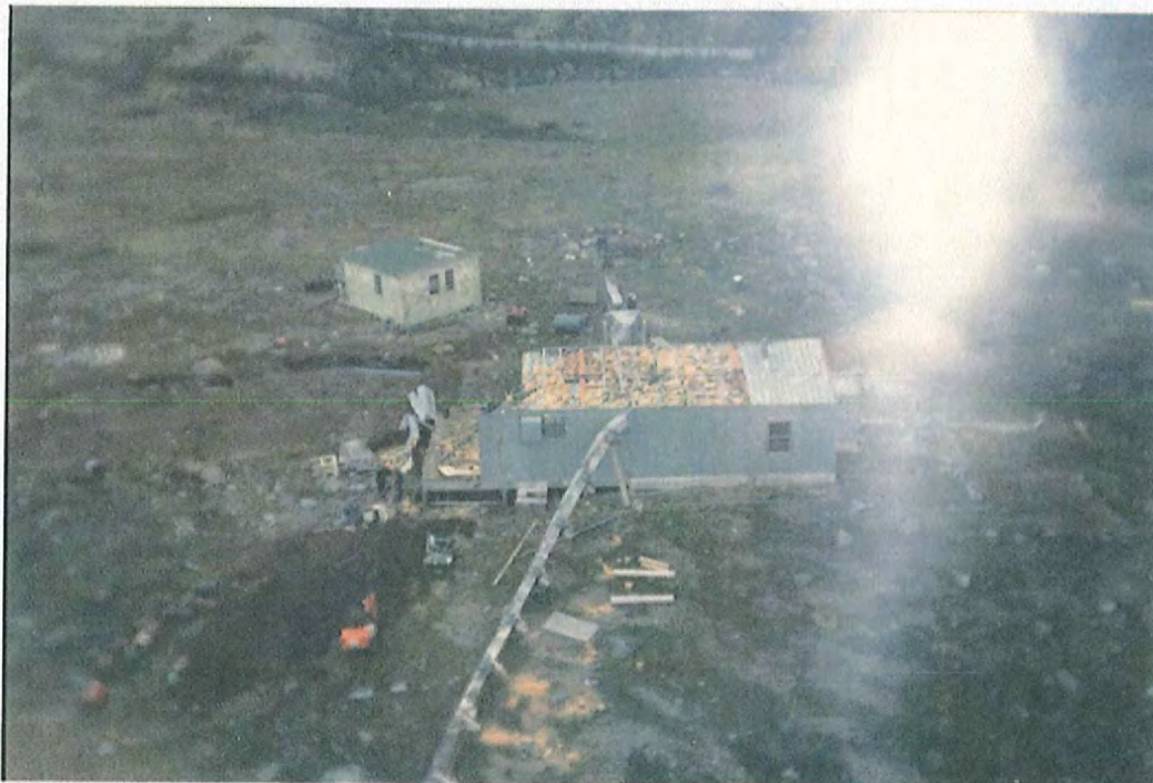
Photo # 2: Site 109 Upper. Demolition in progress.
