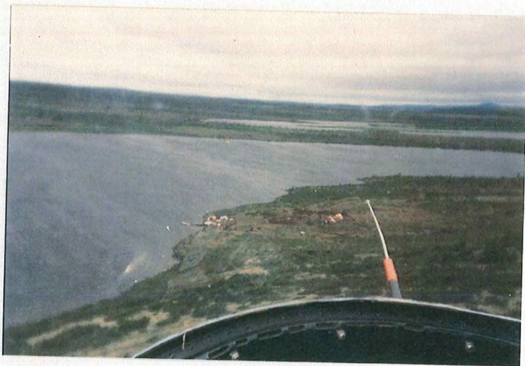
209 Photo # 7: Site 109 Lower. Aerial view of final stages of the work.
