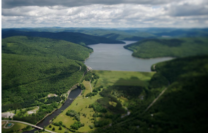
Pepacton Reservoir, Downsville, NY
