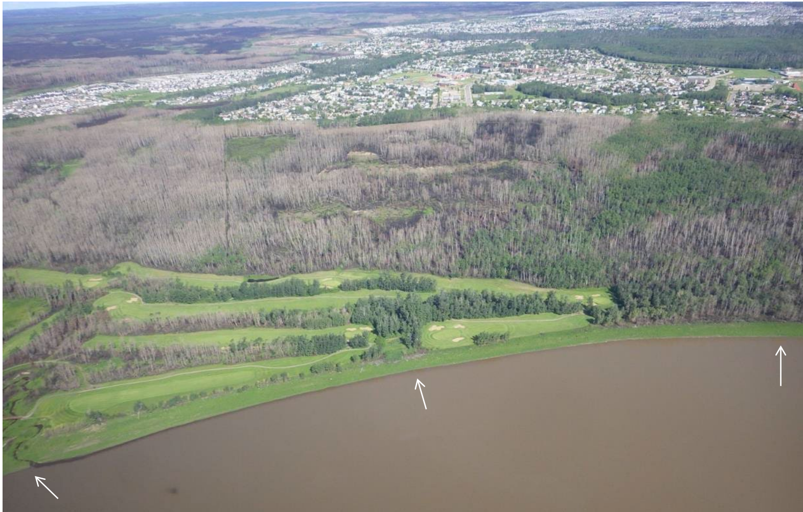
Little Fisheries Creek Upstream of FMM WTP
