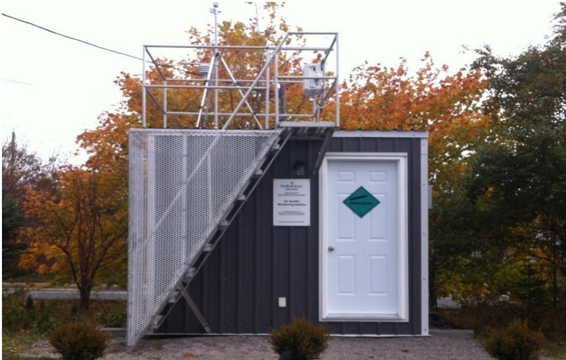
NAPS monitoring station in Mt. Pearl
