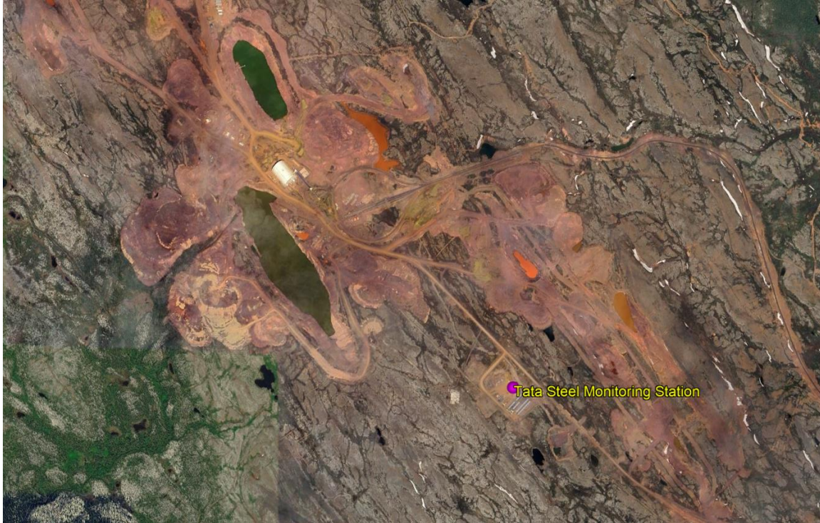
FIGURE 4.10.1 - TSMC AIR QUALITY MONITORING STATION
