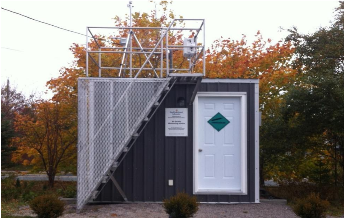
NAPS air quality monitoring station in Mt. Pearl
