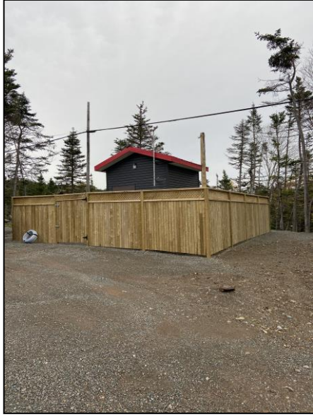
Figure 2: Hut Structure for groundwater well
