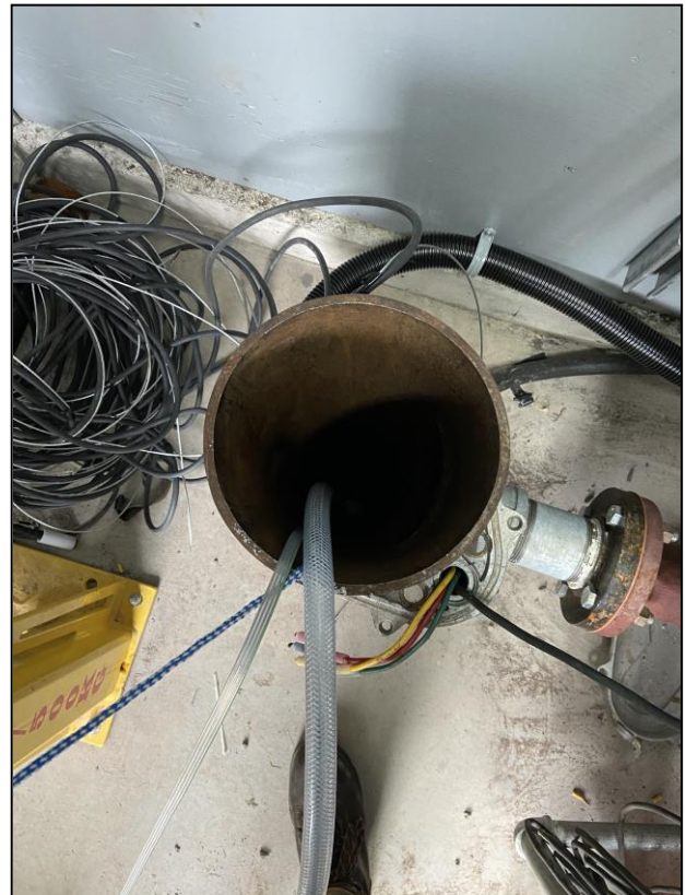
Figure 5: View looking into well
