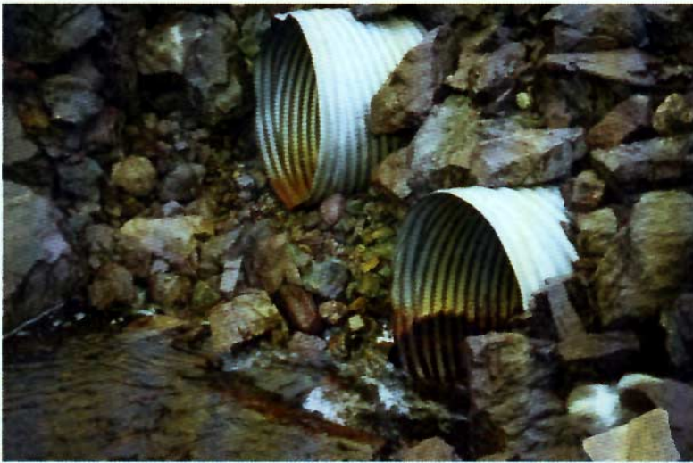
Figure 4.22 Multiple Culvert Installation
