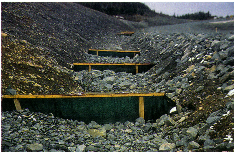
Figure 4.3 Filter fabric dams used in series maximize the effectiveness of the removal of suspended sediment from collected water.
