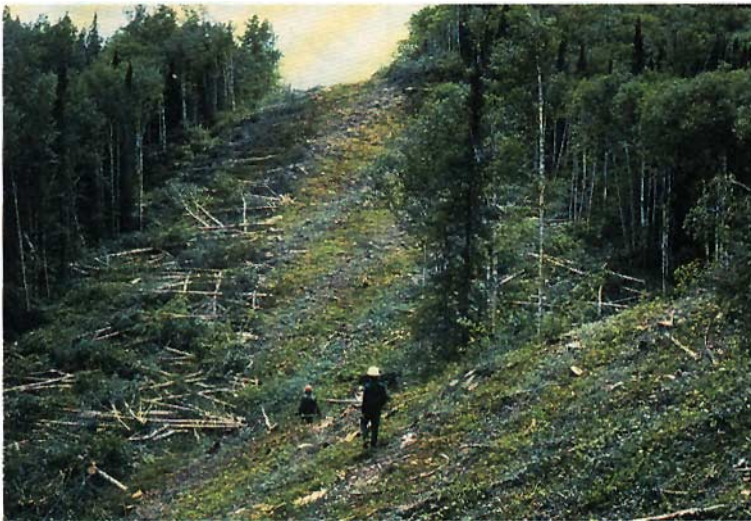
Figure 4.31 Right-of-way clearing and grubbing is commonly associated with many construction developments, including roads, pipelines and transmission lines.
