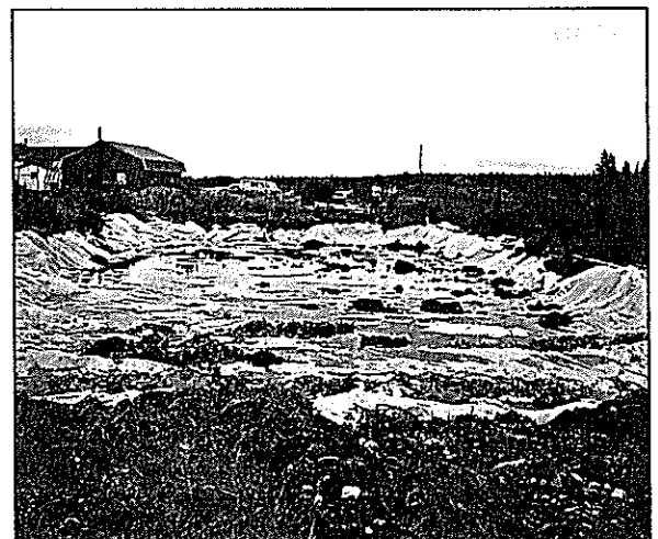
Settling basin lined with plastic.
