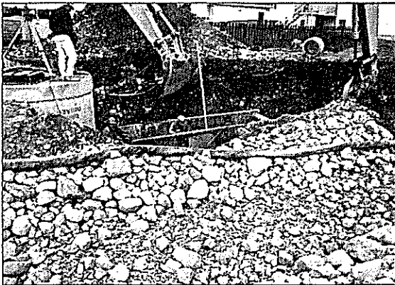
Stream bed restored.
