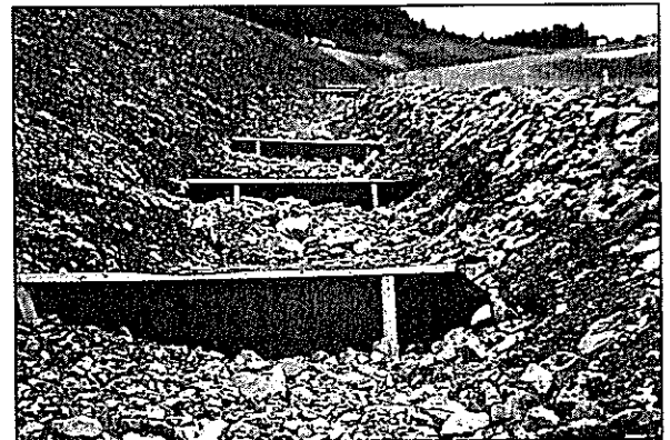
Filter fabric used for low point protection.
