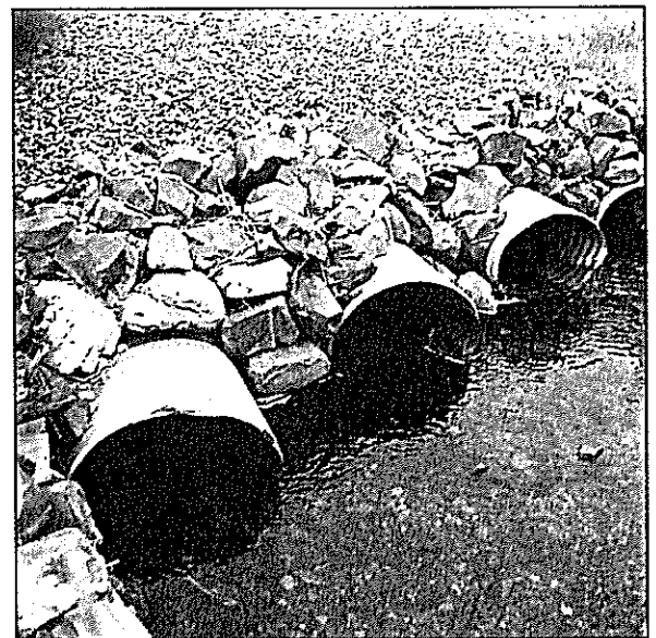
Stabilization of culvert outlets - rip rap.
