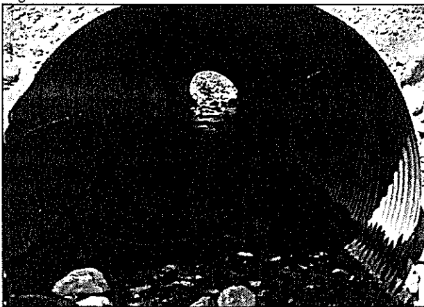
Figure 3. Countersunk Culvert
