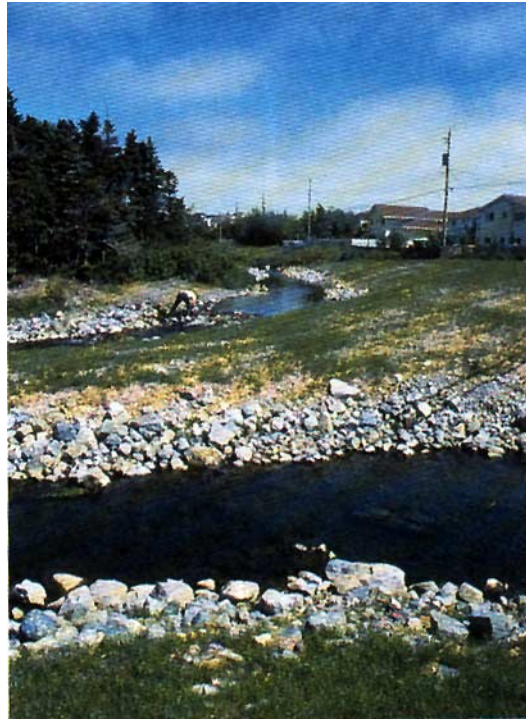
Figure 4.14 Rock riprap prevents erosion.
