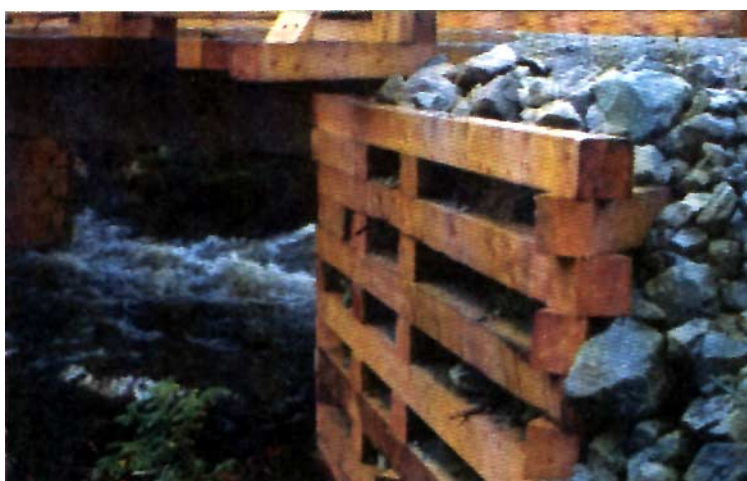
Figure 4.15 Infill materials for timber cribs should be blocky, angular and free of fines or sediment.
