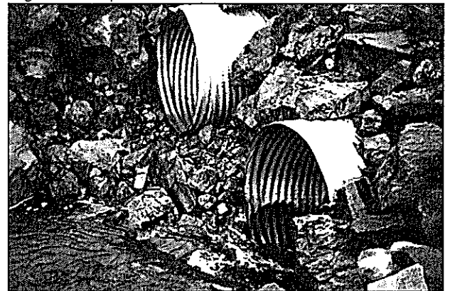
Figure 4. Multiple Culvert Installation
