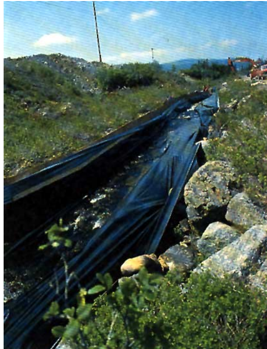
Figure 4.35 Temporary diversion channels should be lined with plastic that is weighted down with stone.
