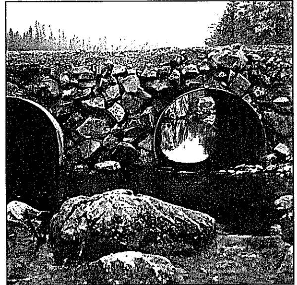
Culvert rip rap stabilization.
