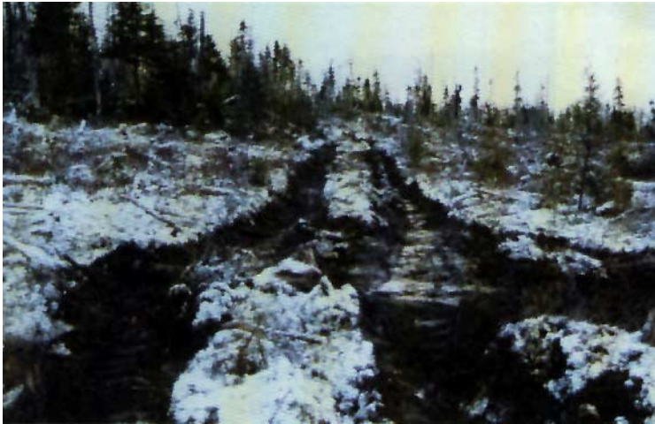
Figure 4.42 Mudlogs divert water off of the trail and onto the forest floor.
