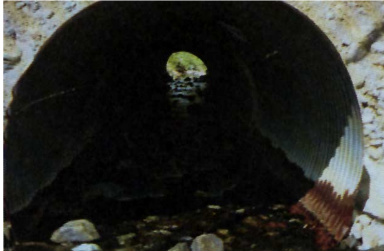
Figure 4.21 Countersunk Culvert.
