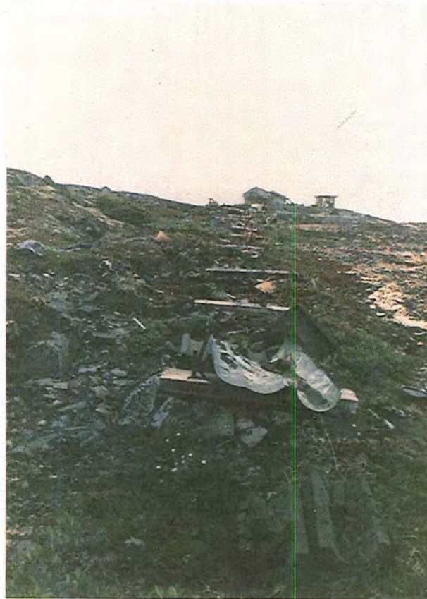
Photo #5: Water Pipeline "Aillik"
