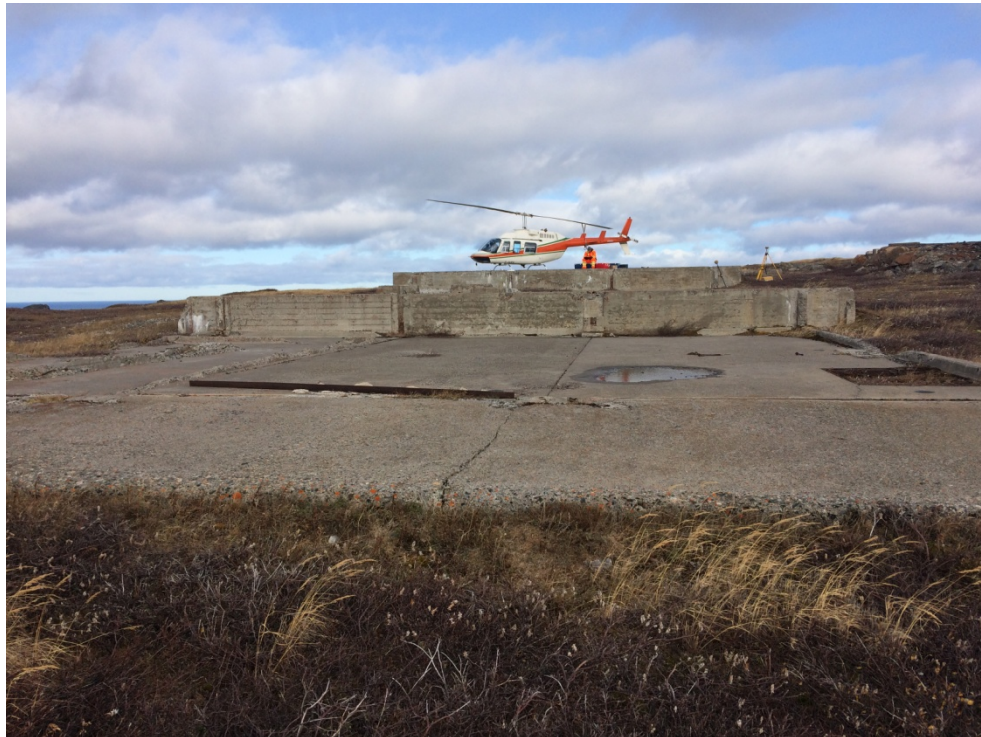
Photo 6: (Upper Site) Foundation of Former Barracks Looking North
