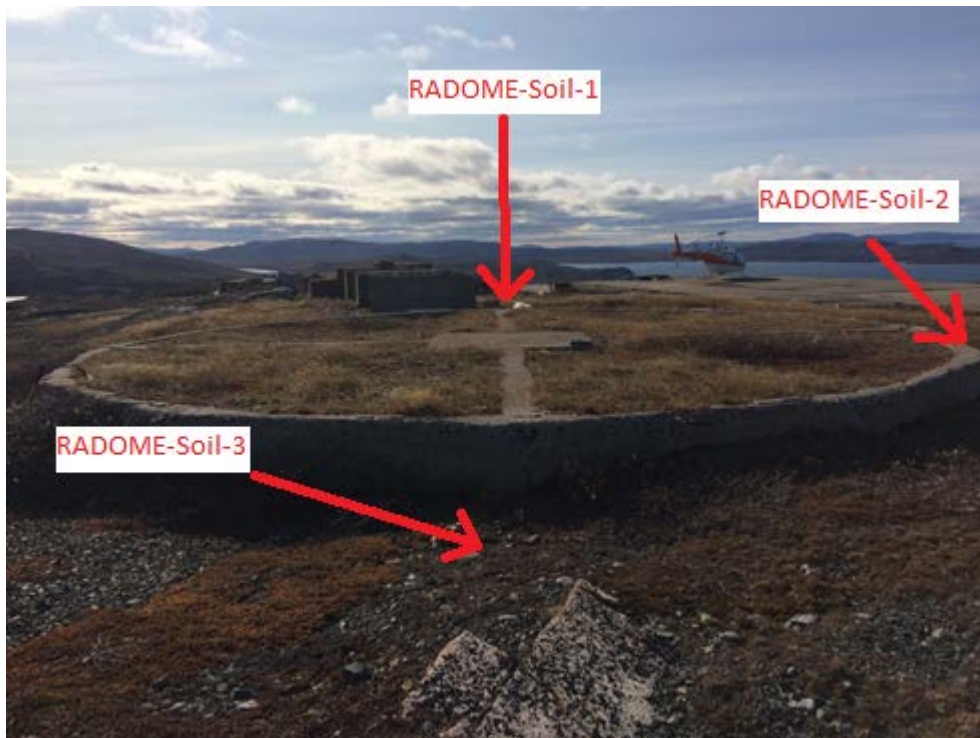
Photo 8: (Upper Site) Foundation of Former Towers looking North
