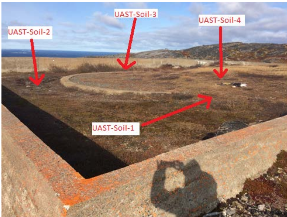
Photo 3: (Upper Site) Concrete Dyke for Former AST Looking North
