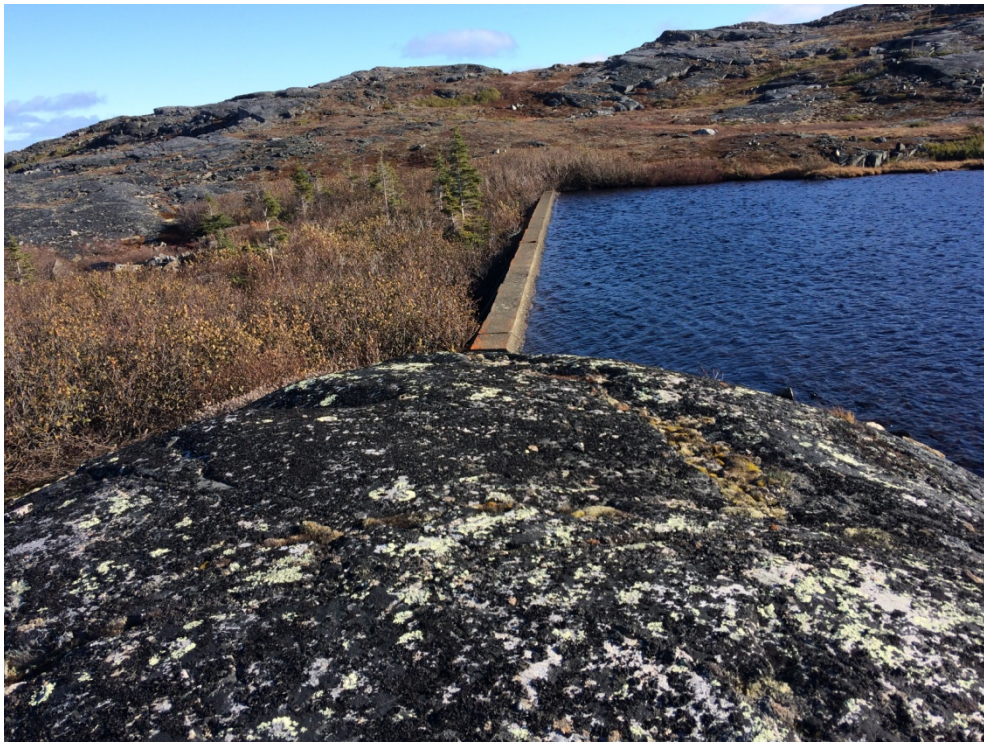
Photo 29: Concrete Dam at Former Water Supply Pond
