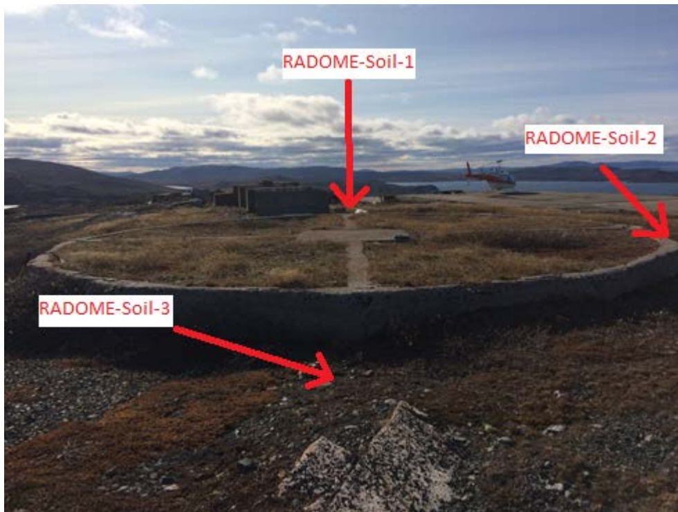
Photo 7: (Upper Site) Foundation of Former Radome Looking West
