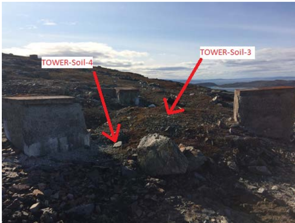
Photo 9: (Upper Site) Foundations of Former Towers Looking West
