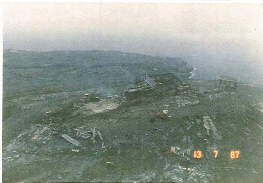
Photo #4: "Aillik" Main Complex Being Dismantled
