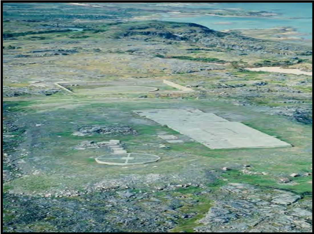
Photo 15: View, looking southwest, towards the concrete remains of the upper Site at Cape Makkovik - July 2002.
