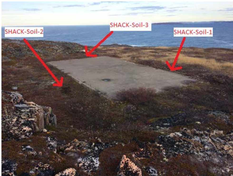
Photo 11: (Upper Site) Foundation of Former Disaster Shack Looking East
