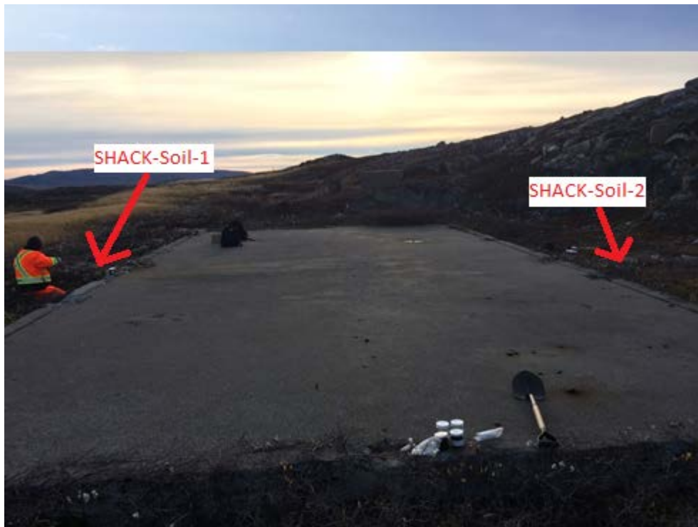
Photo 10: (Upper Site) Foundation of Former Disaster Shack Looking West
