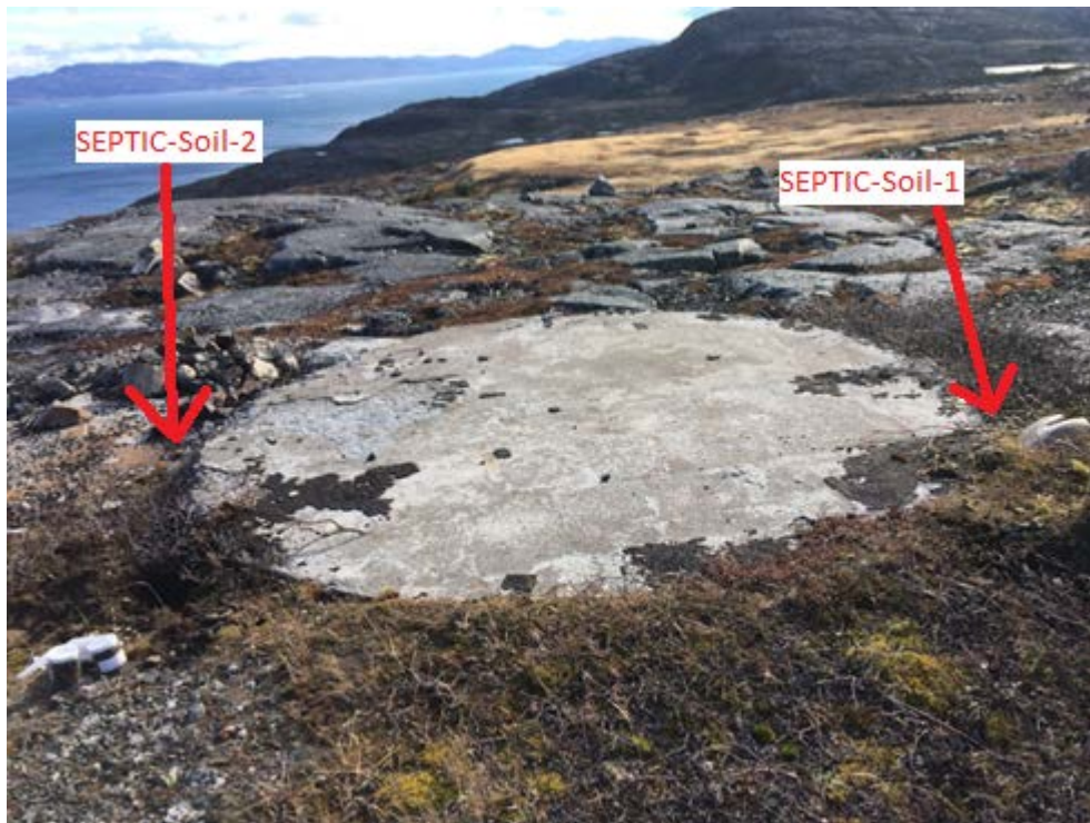
Photo 13: (Upper Site) Foundation of Former Septic Tank Looking South
