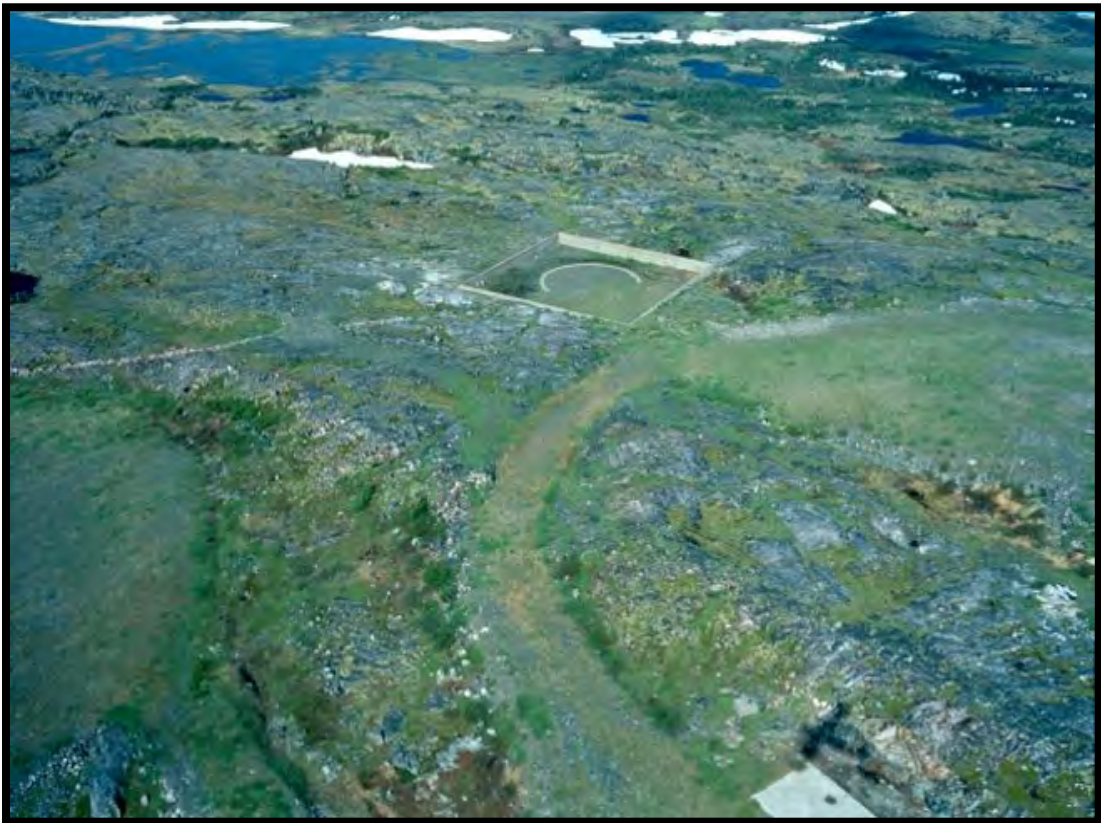
Photo 16: View, looking southwest, towards the concrete remains of the upper Site AST - July 2002. Note the concrete foundation of the disaster shack in the bottom of the photograph.
