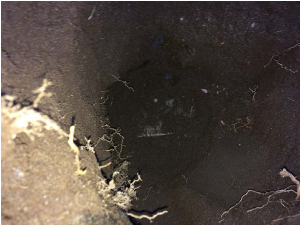
Photo 44: (1987 Disposal Site) Buried building siding and black foam (Sample A1) in test pit where soil sample 1987-SOIL-3 was collected
