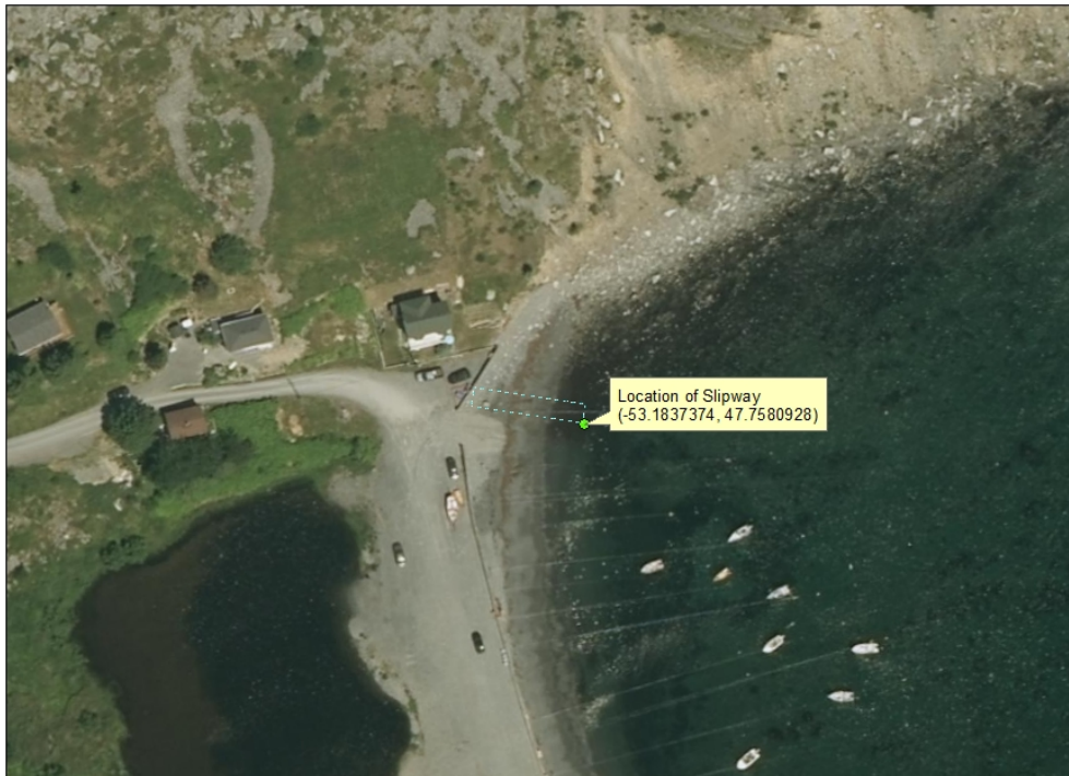
Slipway Construction in the Local Service District of Freshwater
