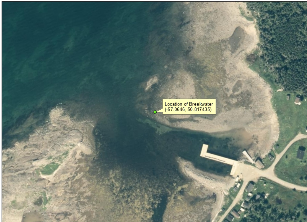
Construction of a Rubble Mound Breakwater in Barr'd Harbour
