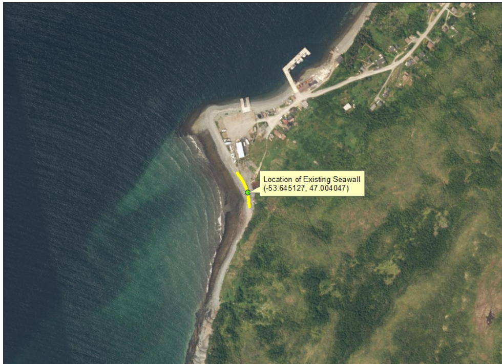
Repairs to a Seawall in the Town of Admirals Beach
