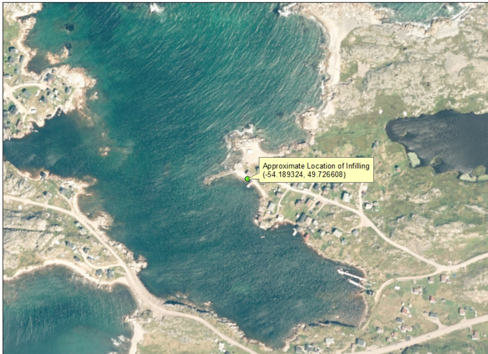
Shoreline Protection at 3 Hewitt's Point Road in the Town of Fogo Island
