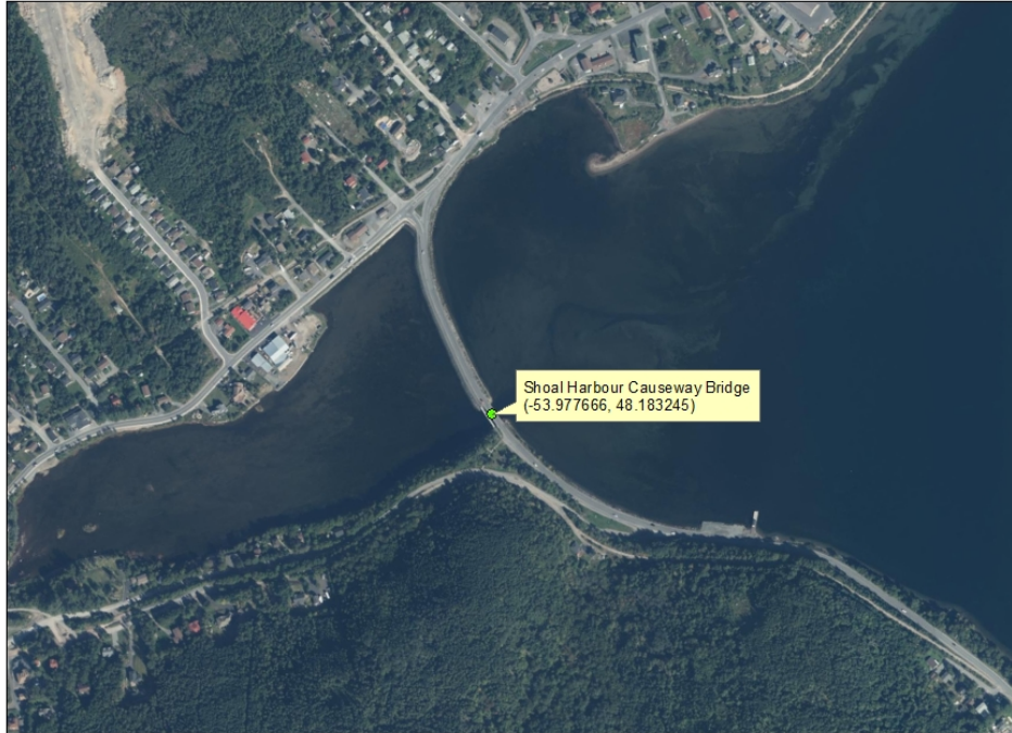
Shoal Harbour Causeway Bridge Replacement in Clarenville
