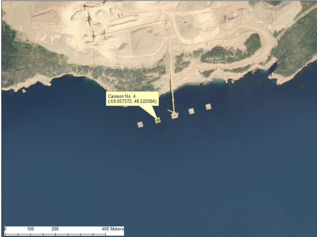
Atlantic Minerals Limited Marine Terminal Caisson No. 4 Replacement
