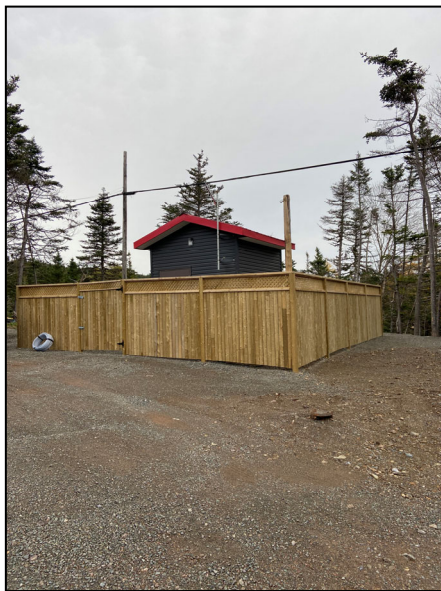
Figure 2: Hut Structure for groundwater well
