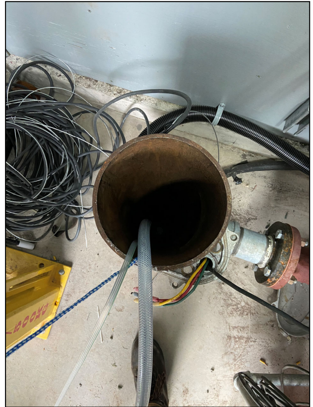
Figure 5: View looking into well
