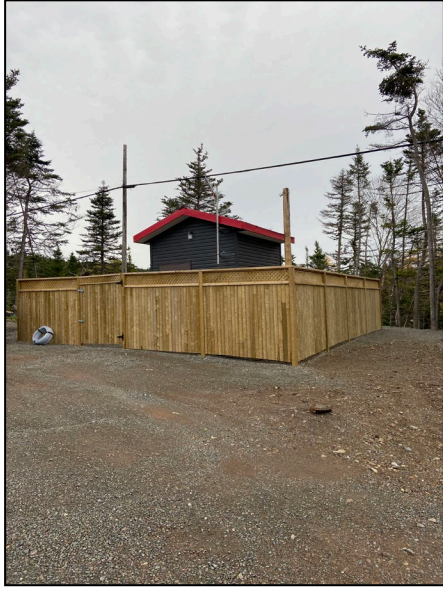
Figure 2: Hut Structure for groundwater well
