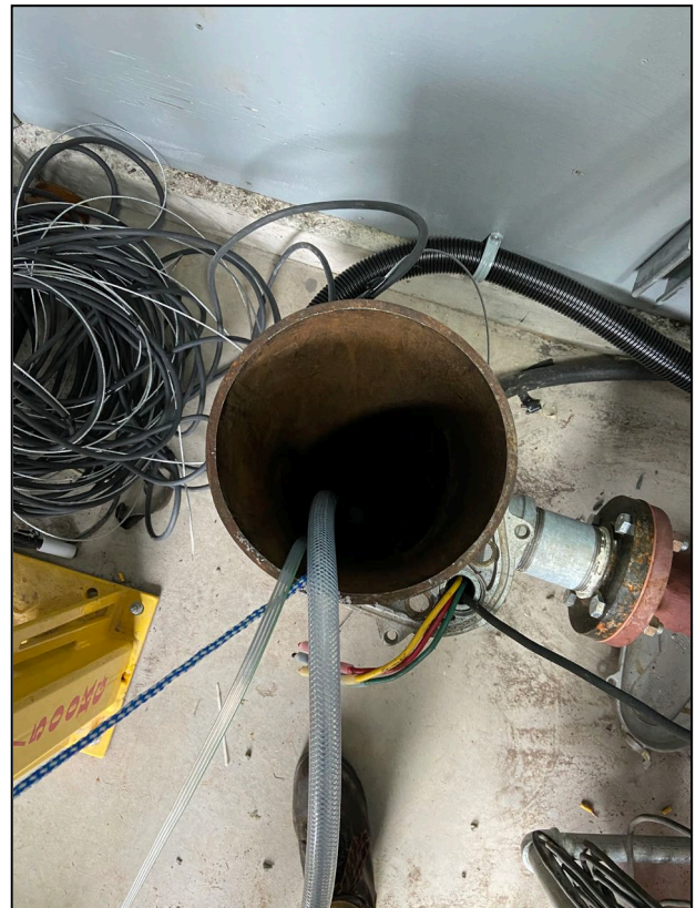
Figure 5: View looking into well
