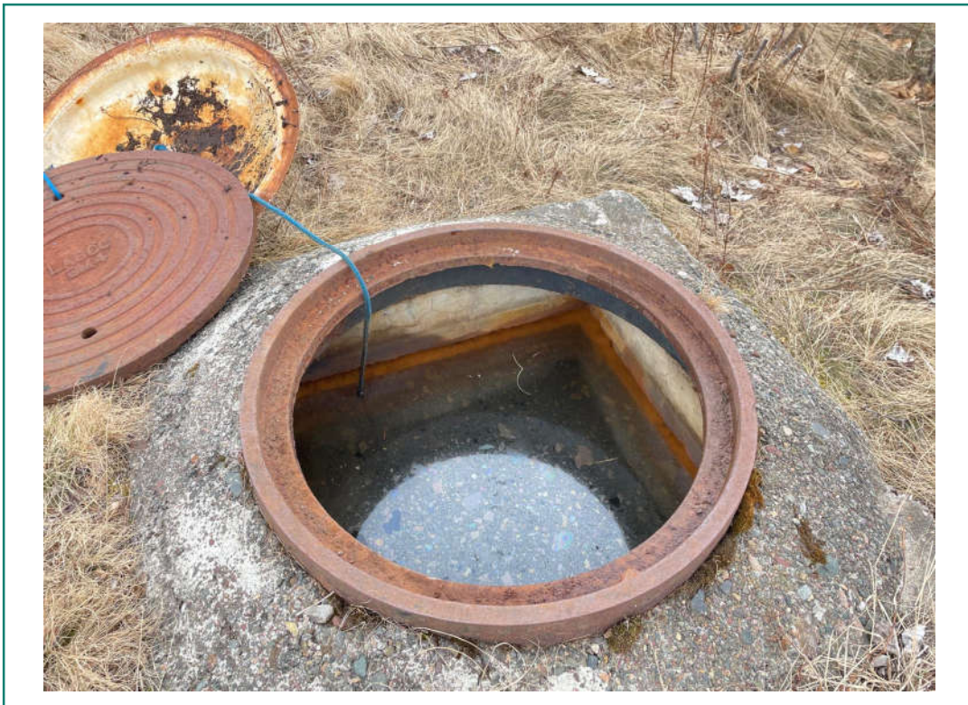
Photo 8: View of the conditions and static water level in the secondary liner containment system (SLCS).
