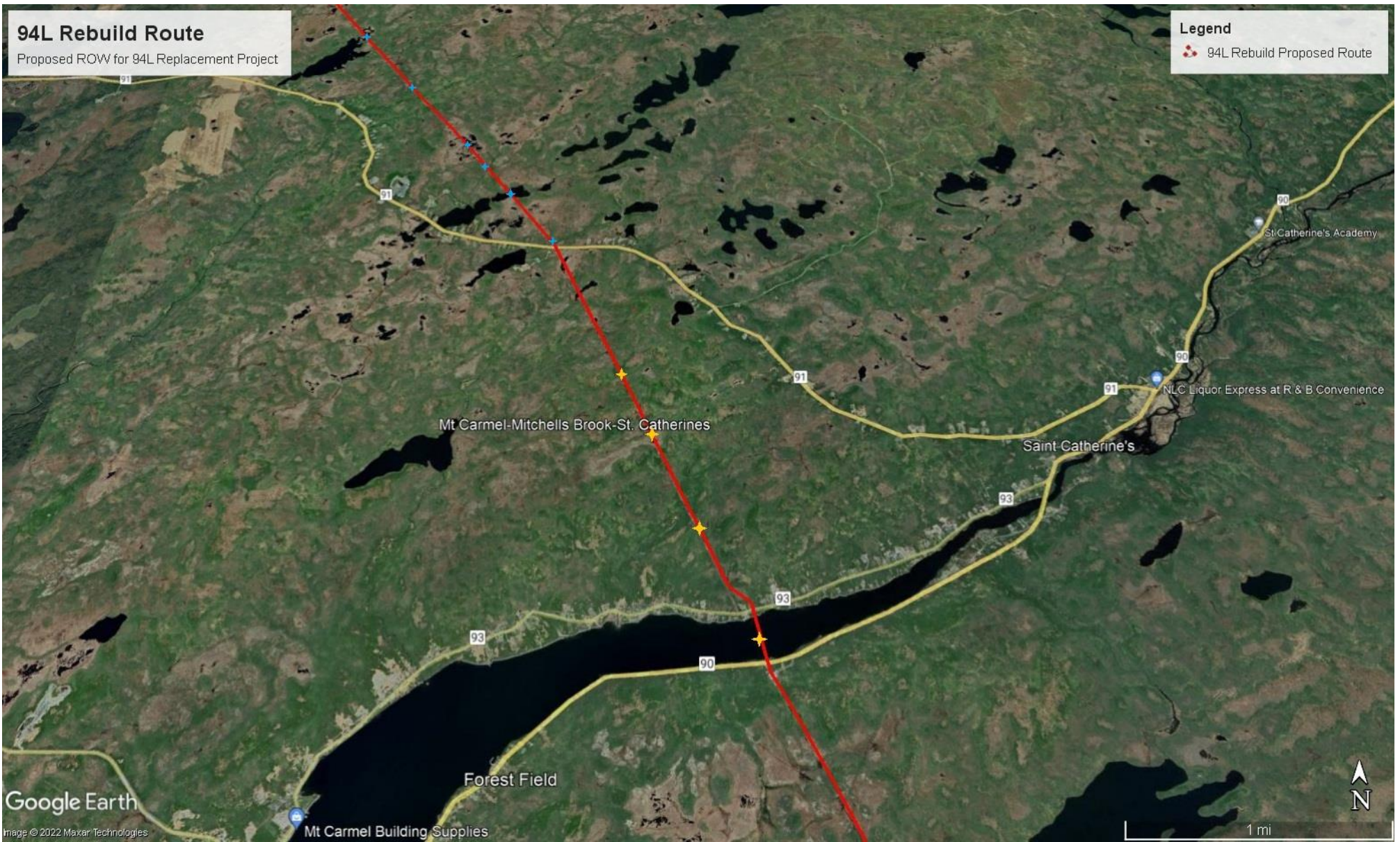
Figure B-5: Phase 2 (2023) extending from St.Catherine's Substation approximately halfway to Blaketown Substation. Crossing sites of rivers identified on 1:50 000 mapping are identified by a blue marker. Crossings of Salmon rivers and tributaries identified on 1:50 000 mapping are identified by a yellow marker.
