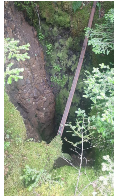
Allow for safe access to the mine shafts.
