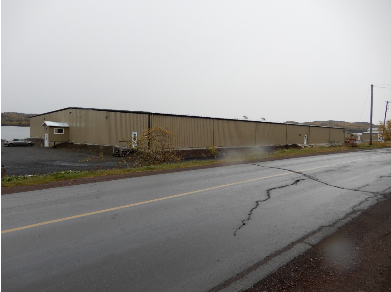
Superior Glove - Pt Leamington Location - Prefabricated Steelway Building
