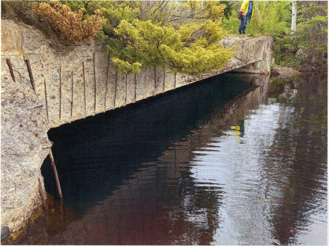
Fig. 5: Little Junction River Bridge
