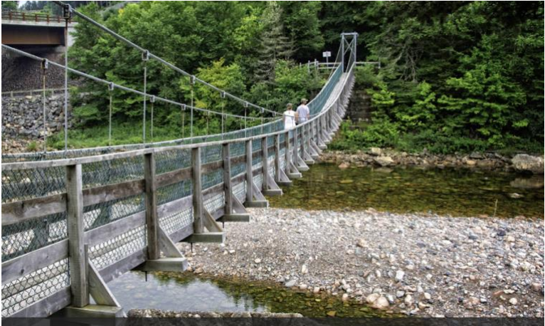
Suspension Bridge to the island
