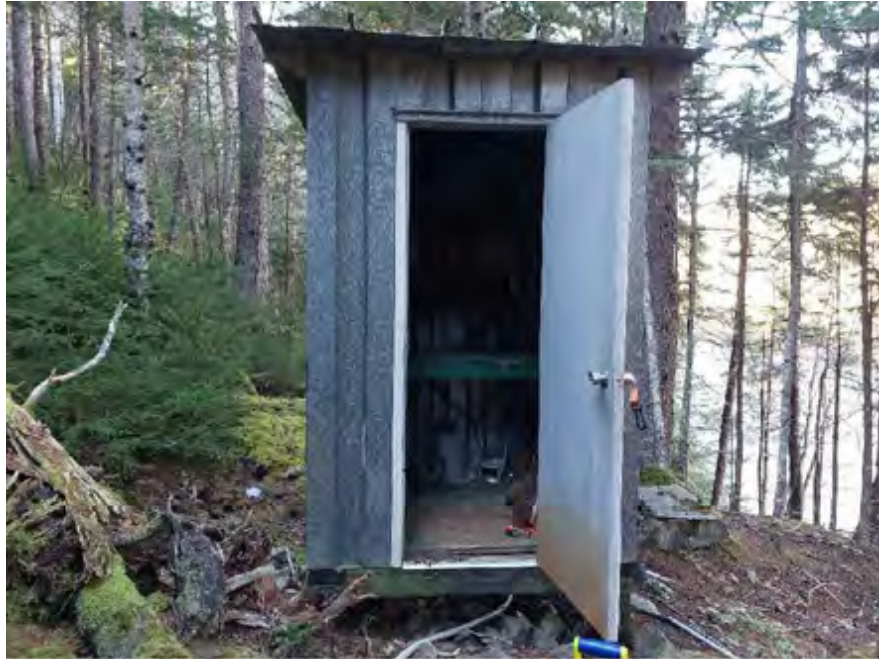
Figure 27. Shelter containing the equipment for the pressure system. Photograph taken mid-November, 2021 (GHD, 2022d).
