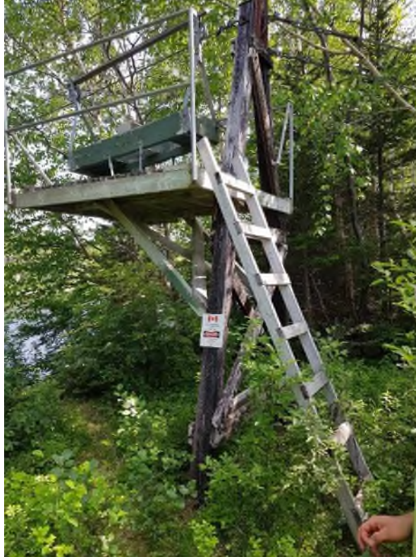
Figure 65. Creosote-treated wooden cableway at 02YS005 Terra Nova River at Glovertown on left bank of the river (photograph taken July 17, 2019).
