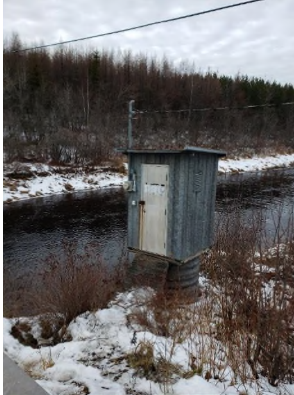
Figure 8. Gauge house and stilling well at 01BS001 Coal Branch River at Beersville (photograph taken on November 15, 2019).
