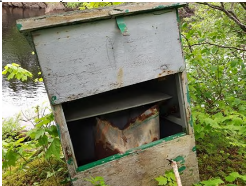
Figure 46. Abandoned stilling well and look-in shelter at 02YC001 Torrent River at Bristol's Pool (Photograph taken July 15, 2019).
