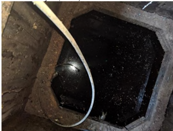
Figure 61. Creosote stave well at 02ZK001 Rocky River near Colinet (Photograph taken on July 18, 2019).
