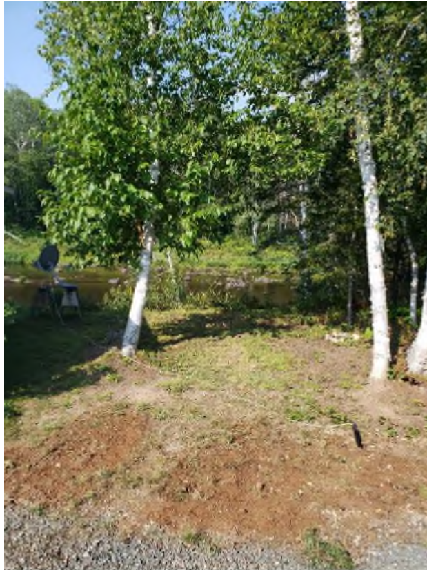
Figure 2. Post construction site at 01BQ001 Northwest Miramichi River at Trout Brook (Photograph August 26, 2021).
