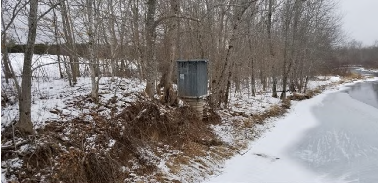
Figure 40. Former stilling well and shelter on left bank of Middle River of Pictou (photograph taken January 28, 2021).
