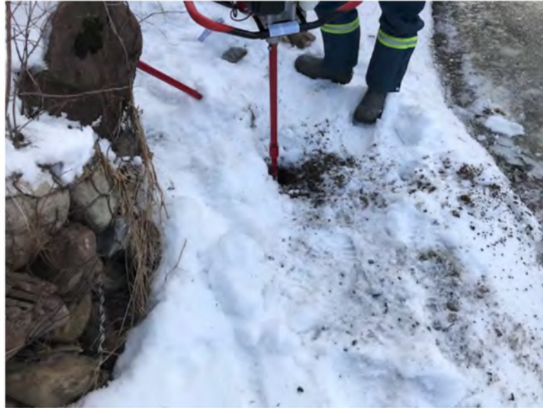
Figure 10. View of power auger used to install monitoring well (MW1) on January 20, 2021 (Photograph from GHD, 2021a).
