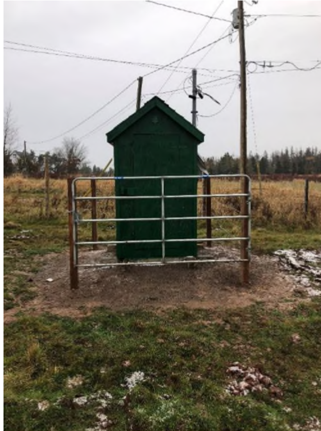
Figure 21. View of shelter after it levelled off and the installation of the fence (photograph taken November 18, 2021).
