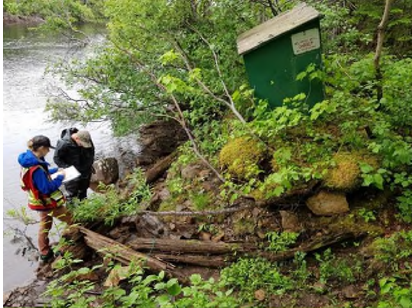
Figure 45. Abandoned stilling well and look-in shelter at 02YC001 Torrent River at Bristol's Pool (Photograph taken on July 15, 2019).
