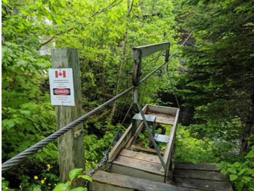
Figure 47. Inactive manned cableway at 02YC001 Torrent River at Bristol's Pool (Photograph taken July 15, 2019).
