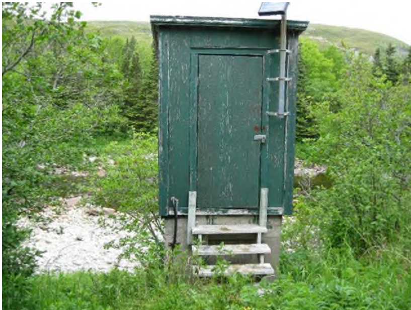
Figure 50. Walk-in shelter above the concrete stilling well at 02ZB001 Isle aux Morts below Highway Bridge (Photograph taken June 21, 2012).
