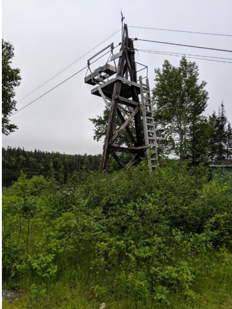
Figure 57. View of former creosote treated timber cableway A-frame and platform located on the left bank of Exploits River (photograph taken July 17, 2019).
