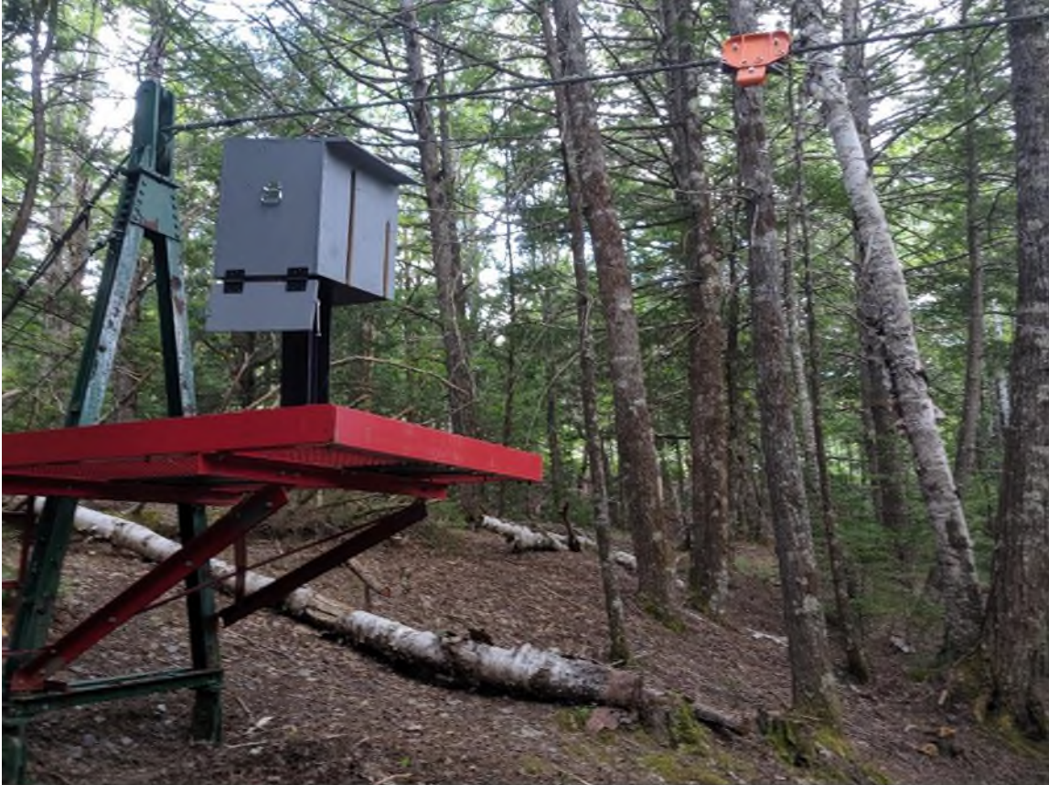
Figure 35. View of the cableway at 01ED007 on the left bank of Mersey River (photograph taken August 9, 2020).
