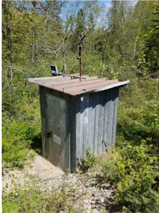
Figure 3. Gauge house and stilling well at 01BP002 Catamaran Brook at Repap Road Bridge (Photograph taken June 6, 2020).
