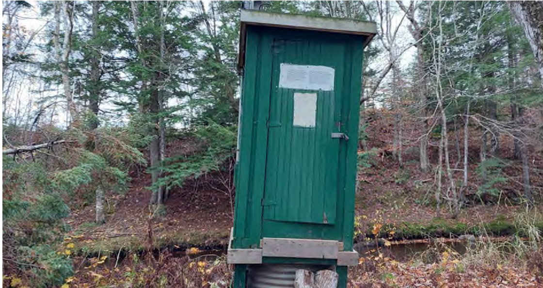
Figure 44. Tilting shelter located at 01AC003. Photograph taken late-October, 2021 (GHD, 2022c).
