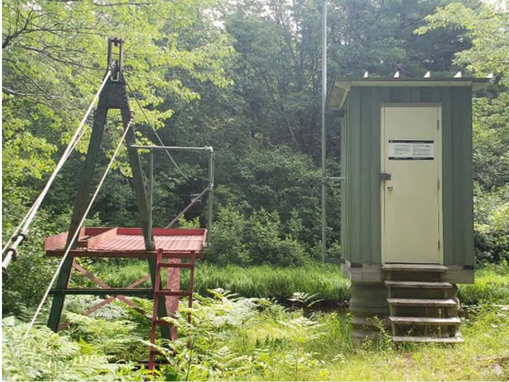
Figure 33. Shelter and an A-frame of the cableway on the left bank at 01DL001 (photograph taken July 22, 2020).
