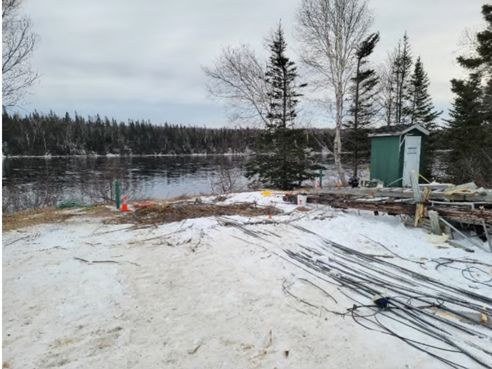
Figure 58. View of cableway decommissioning on the left bank (photograph taken February 22, 2022).
