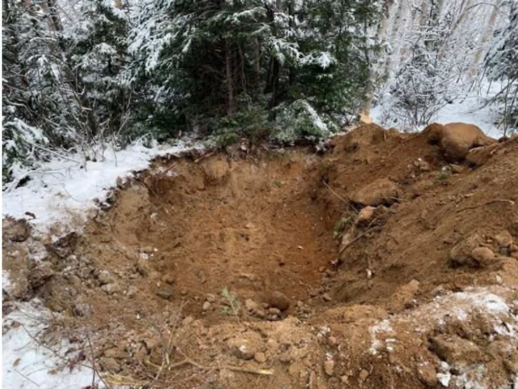
Figure 67. View of the location that the PAH contaminated soil was excavated (photograph taken January 25, 2022).
