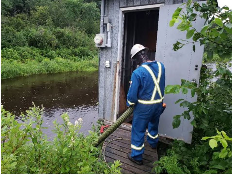
Figure 12. View of well water and sediment being pumped out (photograph taken July 22, 2021).
