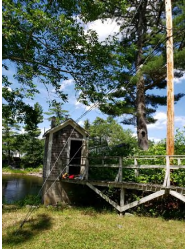
Figure 29. The stilling well and walk-in gauge house at the inactive station 01EE001 Medway River at Charleston (Photograph taken on July 21, 2020).
