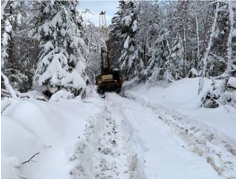
Figure 49. Drill rig entering the site. Photograph taken December 2020 (GHD, 2021c).
