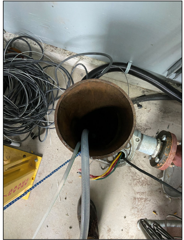
Figure 5: View looking into well
