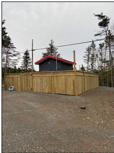
Figure 2: Hut Structure for groundwater well
