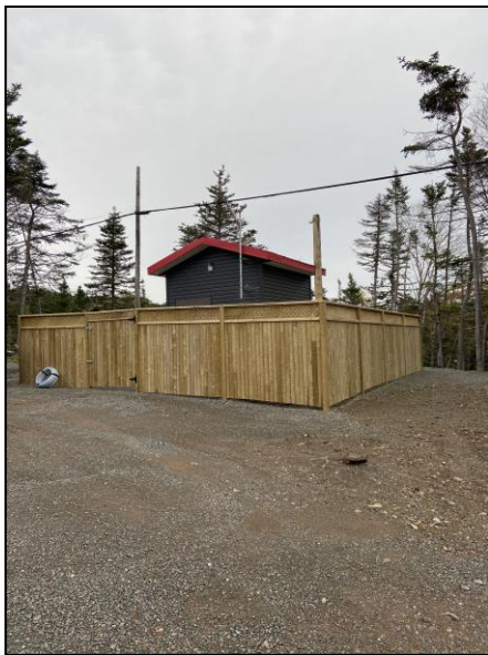
Figure 2: Hut Structure for groundwater well
