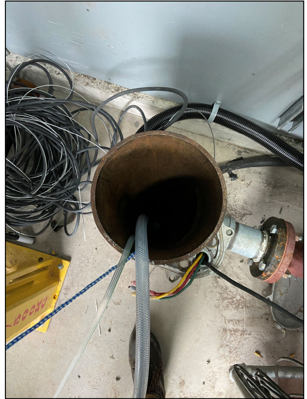
Figure 5: View looking into well
