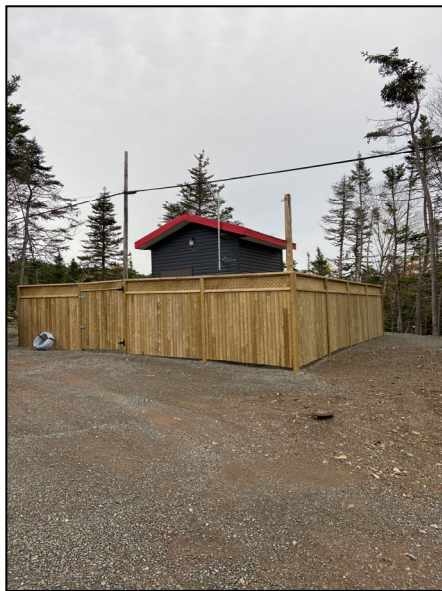
Figure 2: Hut Structure for groundwater well
