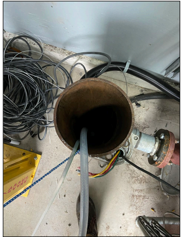
Figure 5: View looking into well
