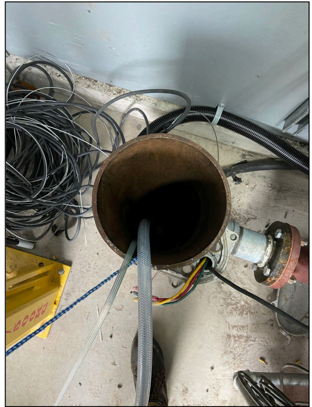
Figure 5: View looking into well
