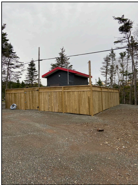
Figure 2: Hut Structure for groundwater well
