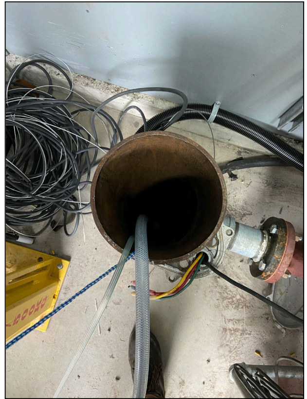
Figure 5: View looking into well
