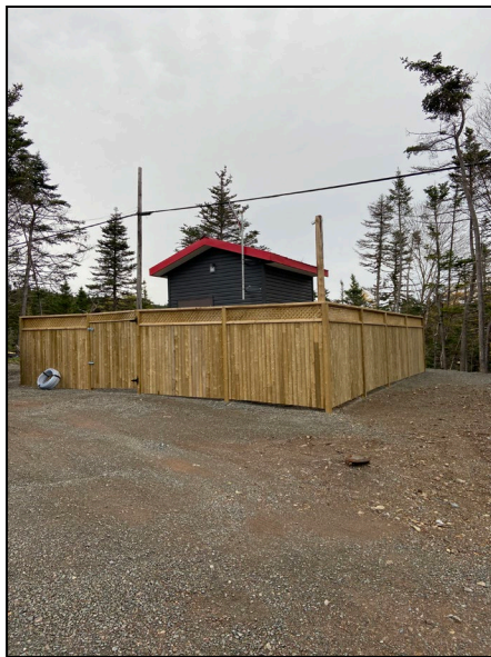
Figure 2: Hut Structure for groundwater well
