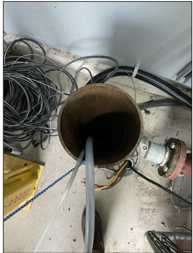
Figure 5: View looking into well
