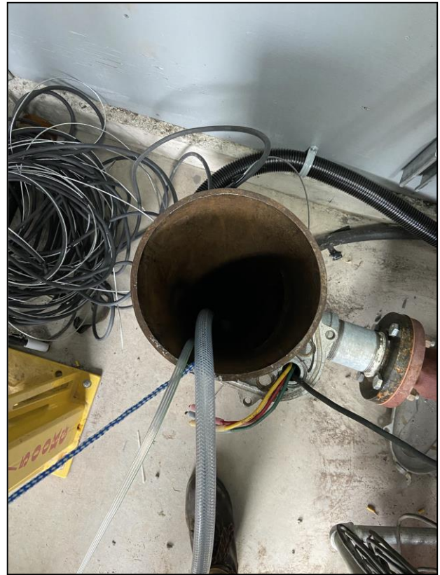
Figure 5: View looking into well
