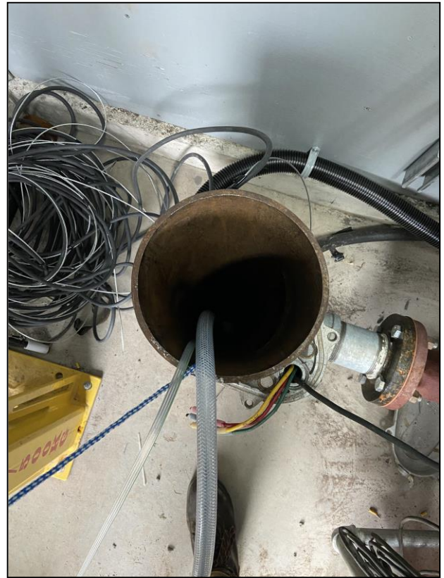
Figure 5: View looking into well
