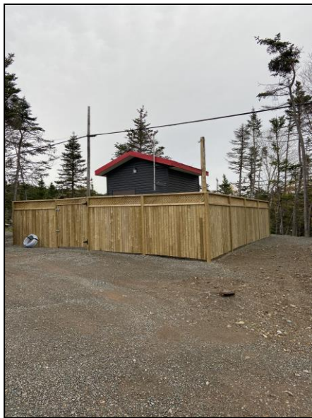
Figure 2: Hut Structure for groundwater well
