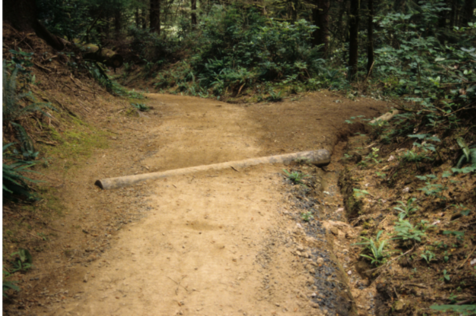
Figure 10 - Photo of installed water bar. (Ebel, 2017)
