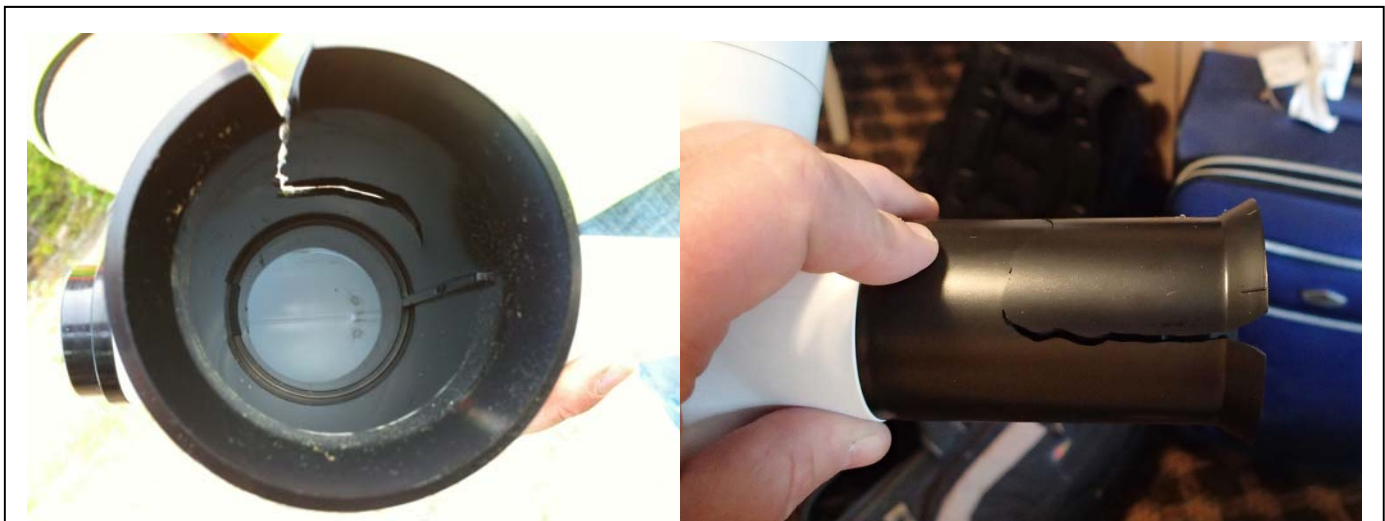
Figure 9: Anemometer housing damage at Churchill River at end of Mud Lake Road
