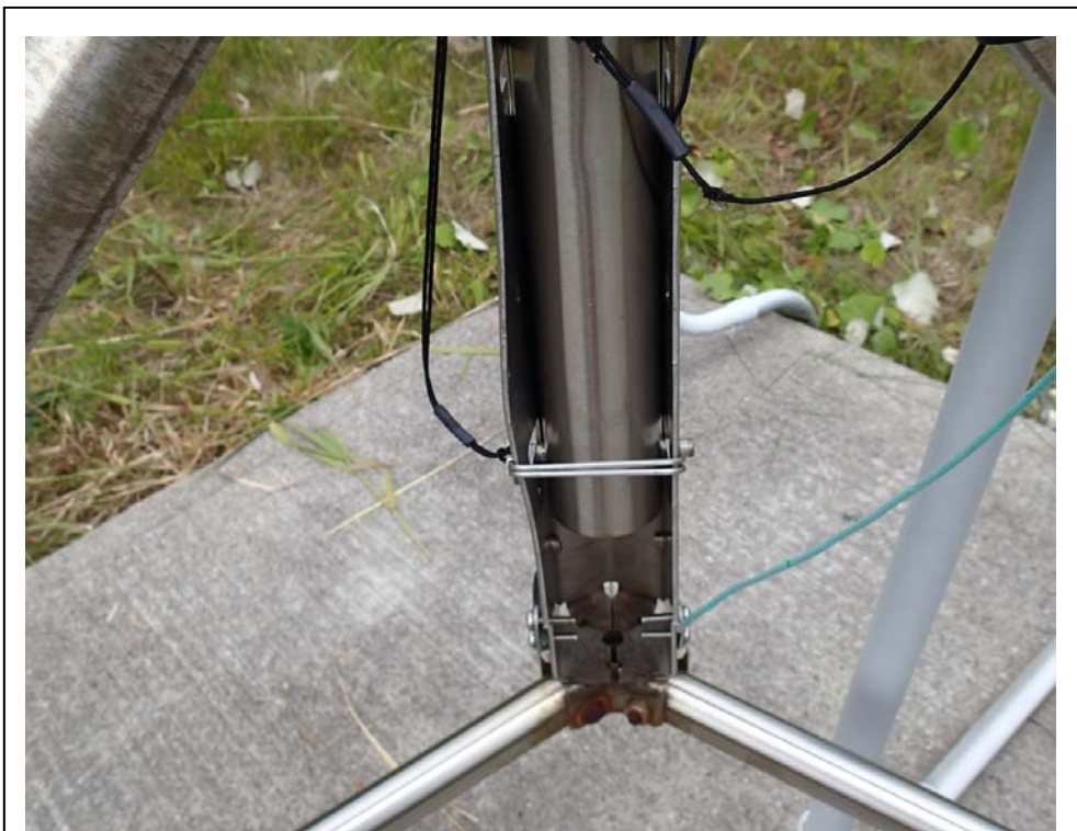
Figure 6: Compromised Tripod Integrity at Humber River At Humber Village Bridge Station
