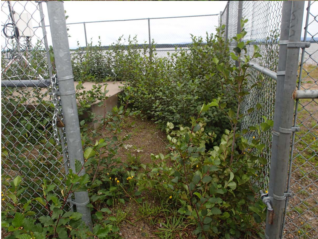
Figure 10: Overgrowth at Churchill River at end of Mud Lake Road
