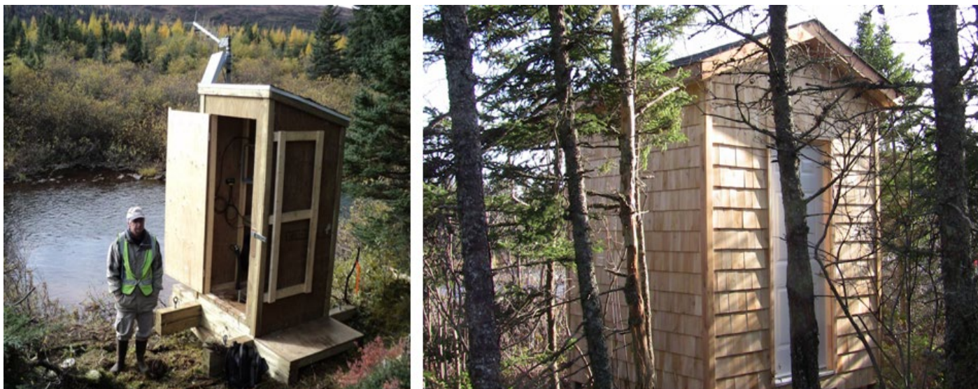
Figure 4-1: (L) Standard design for RTWQ monitoring station; (R) Modified design for RTWQ monitoring test station
