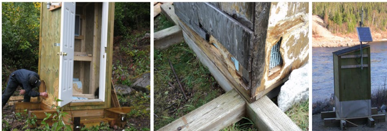
Figure 4-2: (L & M) Animal damage to an RTWQ station on the Churchill River; (R) Metal siding is wrapped around the station shelters to prevent damage by animals
