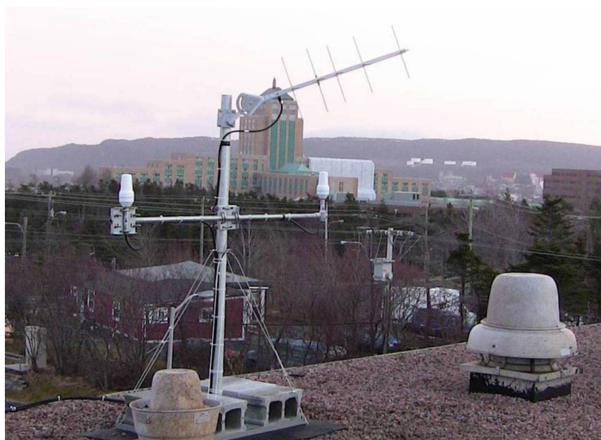
Figure 3-9: Iridium base station located at WRMD headquarters in St. John’s receives data from remote stations
