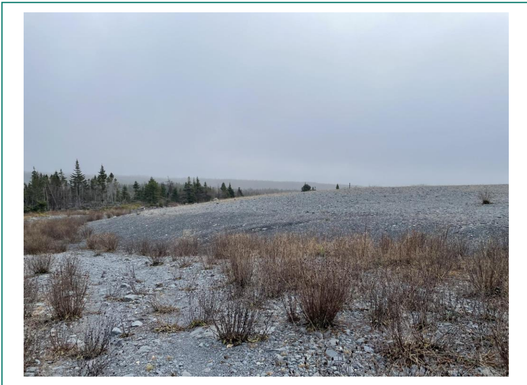
Photo 4: Overview showing current slope conditions of the hazardous waste landfill.
