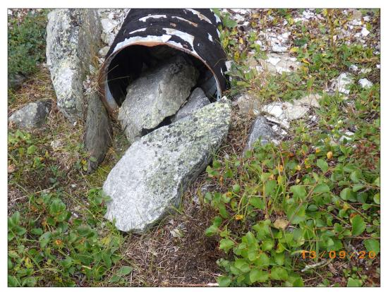
PHOTO 16 - APEC #2: Drain pipe in the berm of the former Lower Site AST. Other black caulking analyzed at the site was found to be asbestos-containing. (September, 2017)
