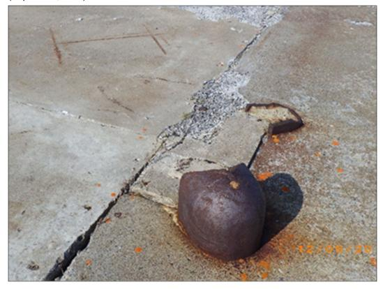
PHOTO 102 - APEC #10: Metal protruding out of the former main building concrete slab. (September, 2017)
