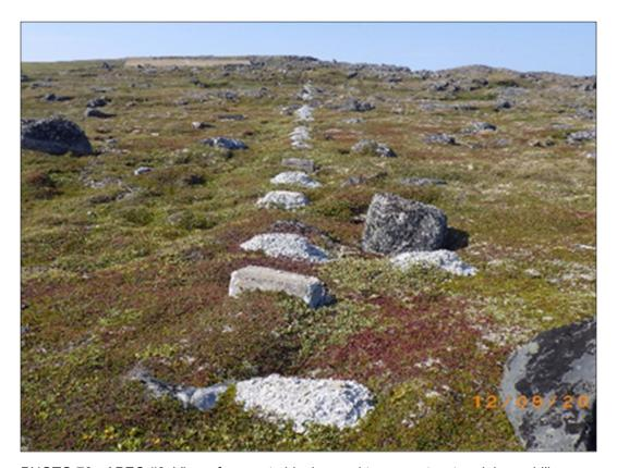
PHOTO 70 - APEC #8: View of concrete blocks used to support water piping uphill. (September, 2017)
