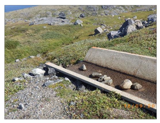
PHOTO 76 - APEC #8: End of concrete drainage channel. (September, 2017)
