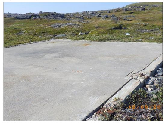
PHOTO 106 - APEC #11: Concrete foundation of former disaster shack. (September, 2017)
