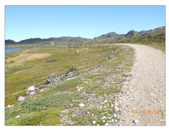
PHOTO 47 – APEC #7: Gravel access road that connects the Upper Site to the lower Site, still in good condition. (September, 2017)
