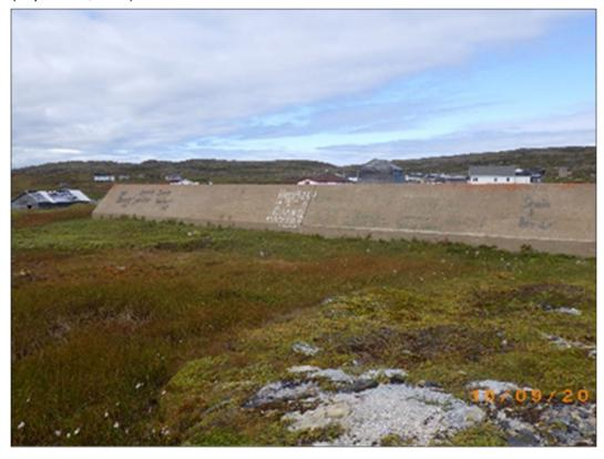
PHOTO 86— APEC #12: Concrete berm around former AST location at the Lower Site. (September 2017)
