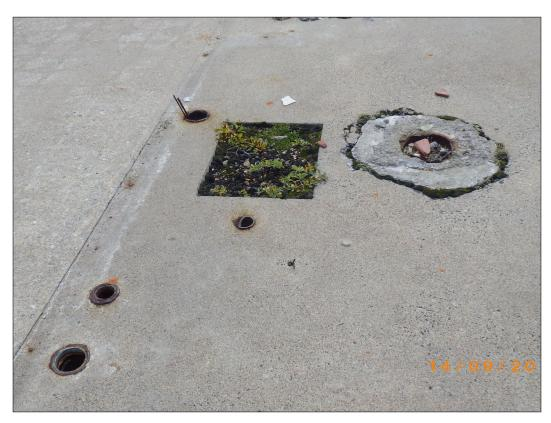
PHOTO 26 - APEC #5: View of penetrations through the slab of the Main building. Metal fittings presumed to be lead-containing. (September, 2017)
