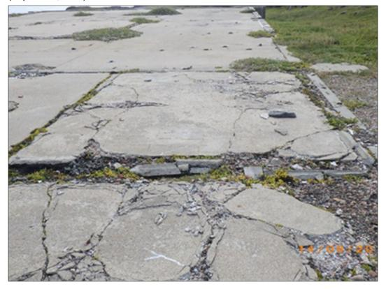
PHOTO 34 - APEC #5: View of former main building concrete slab. Slab is in good condition in most areas, but is degraded in other areas. (September, 2017)
