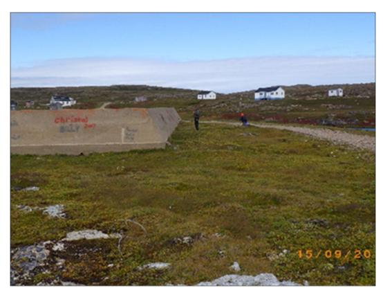
PHOTO 87– APEC #12: Concrete berm around former AST location at the Lower Site, with the gravel access road to the right. (September, 2017)
