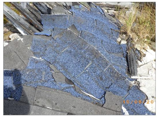
PHOTO 80 - APEC #11: View of asphalt shingles disposed of at APEC #11. (September 2017)
