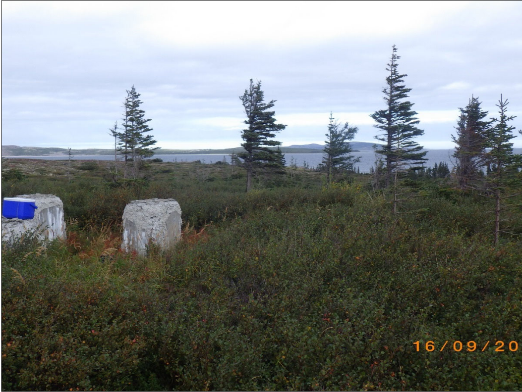
PHOTO 9 - APEC #3: (Former tower structure #1) showing two of the remaining four concrete pillars. (September, 2017)
