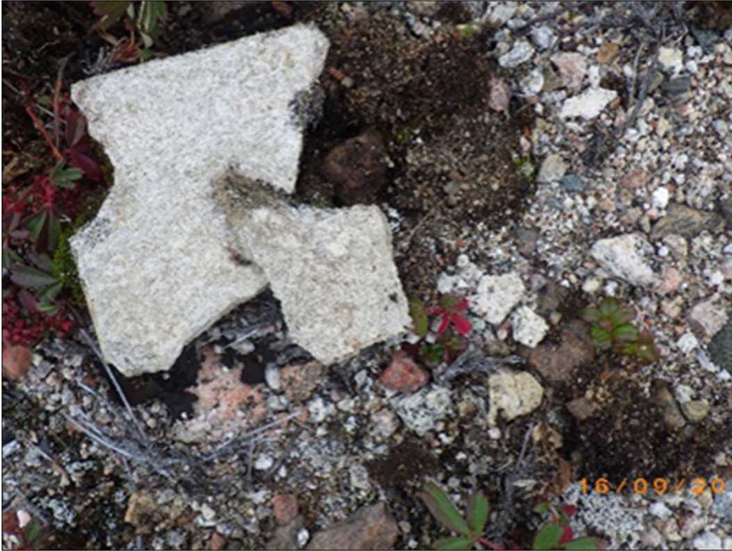
PHOTO 35 - APEC #7: Transite board. (September, 2017)
