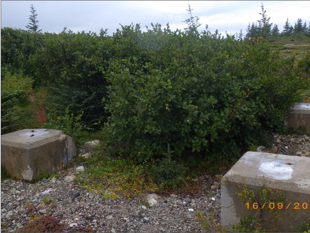
PHOTO 21 - APEC #4: (Former tower structures #2) showing three concrete pillars. (September, 2017)
