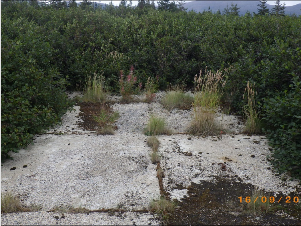
PHOTO 5 - APEC #2: (Former structure) showing remains of concrete foundation. (September, 2017)
