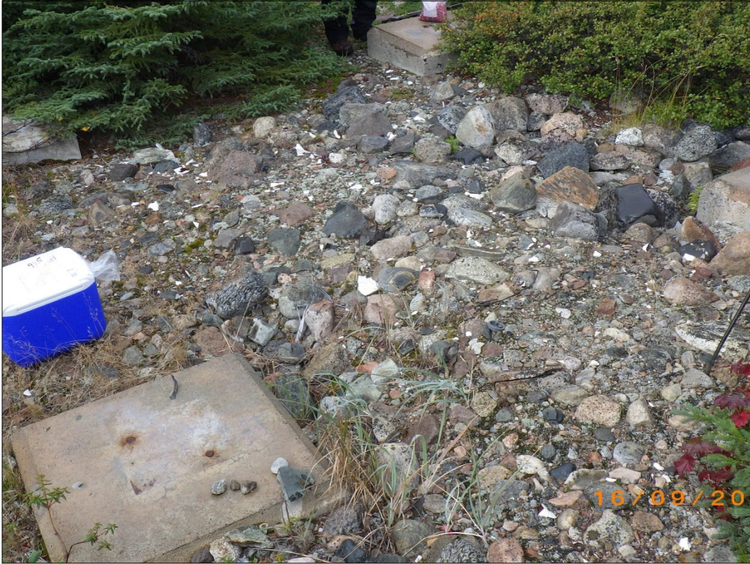
PHOTO 13 - APEC #4: (Former tower structures #2) showing concrete pads. (September, 2017)
