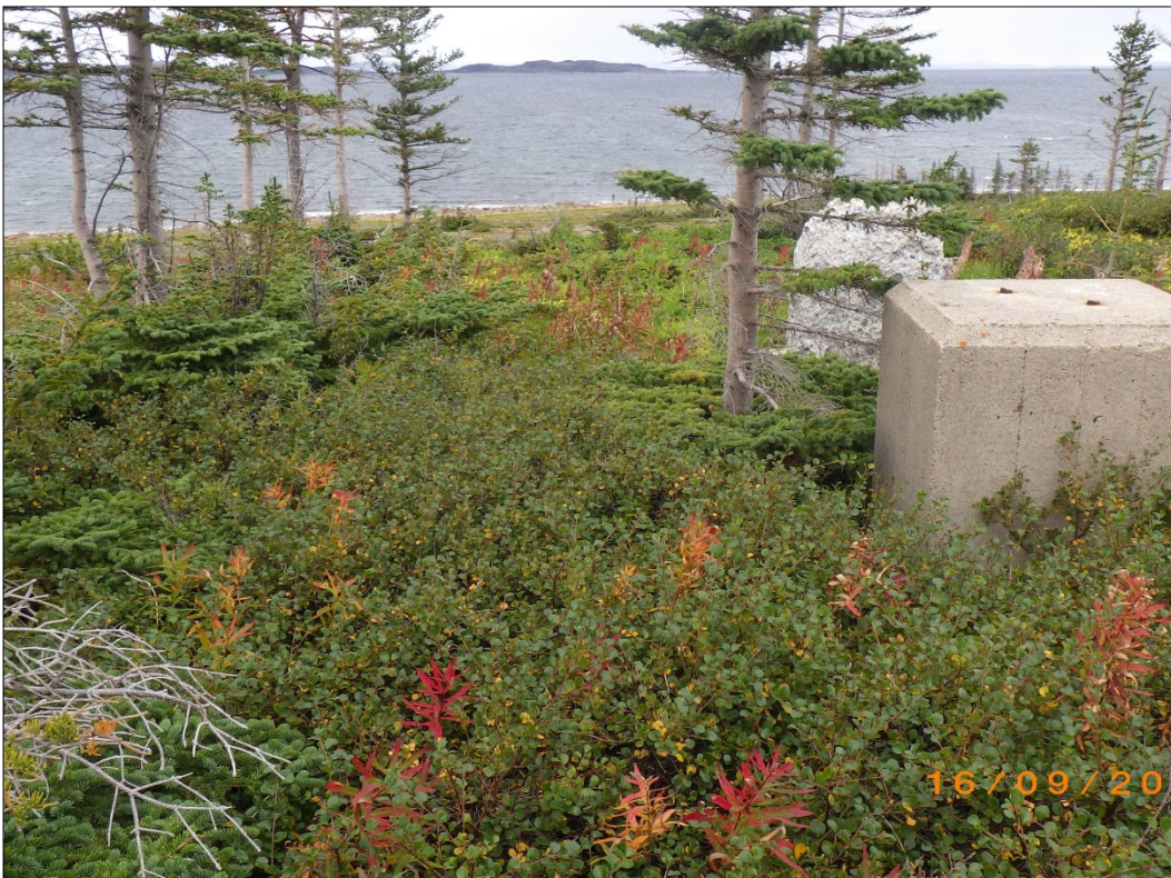
PHOTO 22 - APEC #5: (Former tower structures #3) showing remains of concrete pillars. (September, 2017)
