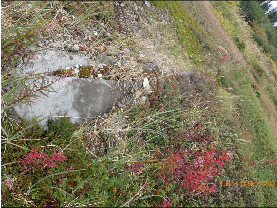
PHOTO 41 - APEC #7: (Presumed landfill) showing buried debris. (September, 2017)
