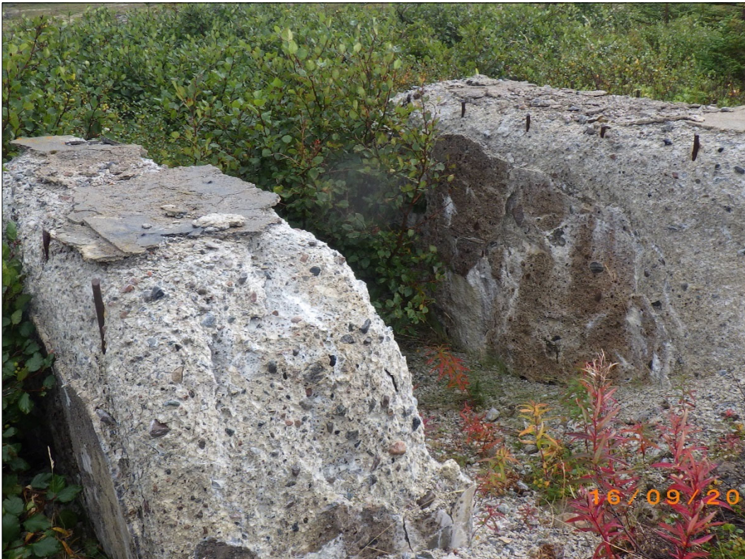
PHOTO 14 - APEC #4: (Former tower structures #2) showing remains of concrete cradle. (September, 2017)
