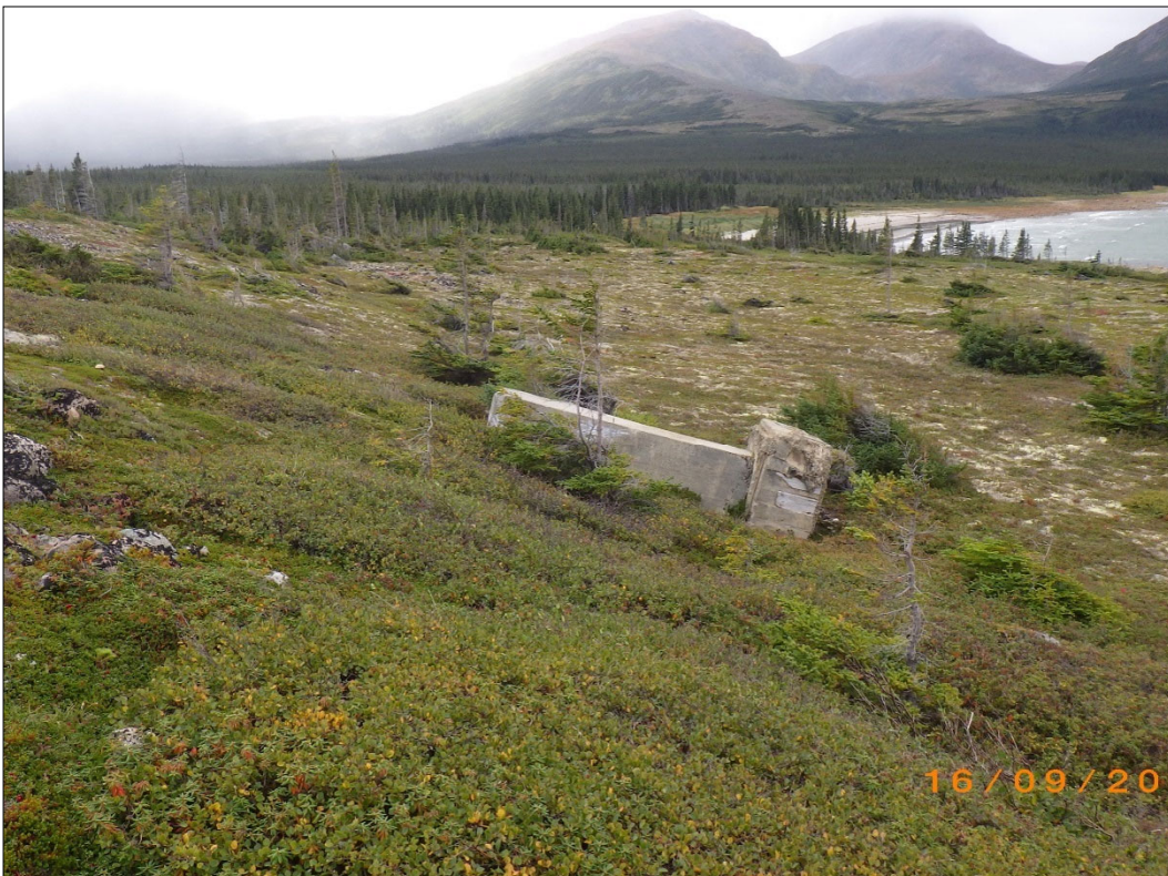
PHOTO 34 - APEC #6: View showing remains of overturned concrete pillars. (September, 2017)
