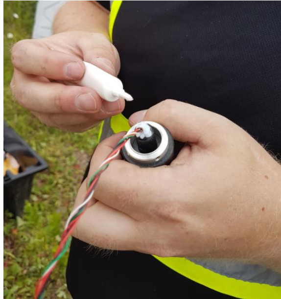
Figure 43: Apply Silicone
