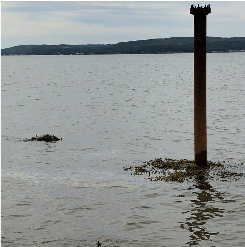
Photo 1 – Oil Sheening near Well Repair #1
