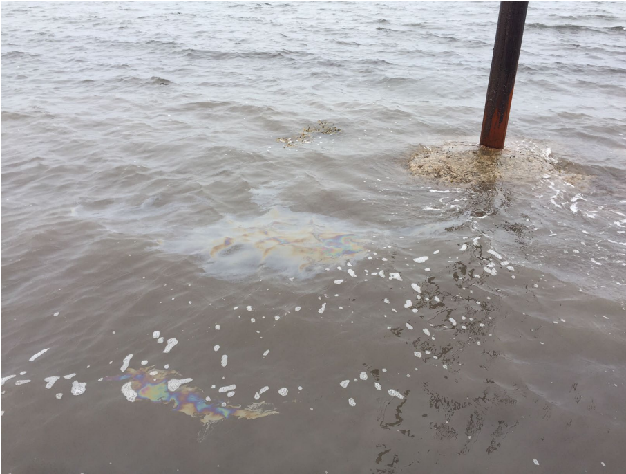
Photo 6 – Oil Seepage/Sheening near Well Repair #1
