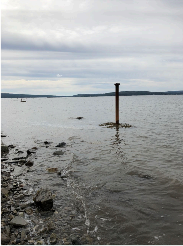
Photo 2 – Oil Sheening near Well Repair #1
