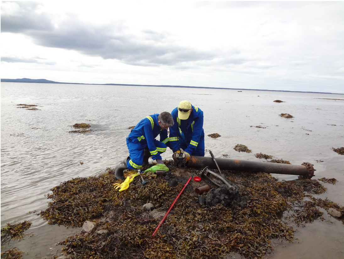
Photo 1 – Plug Installation Well #1
