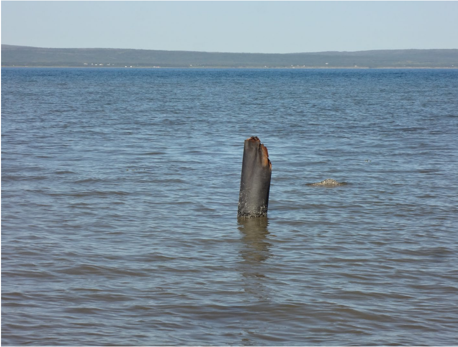
Photo 4 – Abandoned Well Casing
