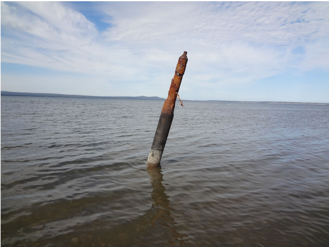
Photo 3 – Abandoned Oil Well Casing (Closest to the Shoal Point Tip)
