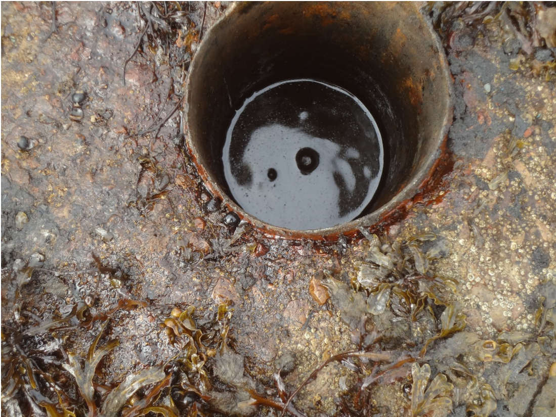
Photo 4 – Oil/Water Accumulation and Gas Bubbles after Plug Installation
