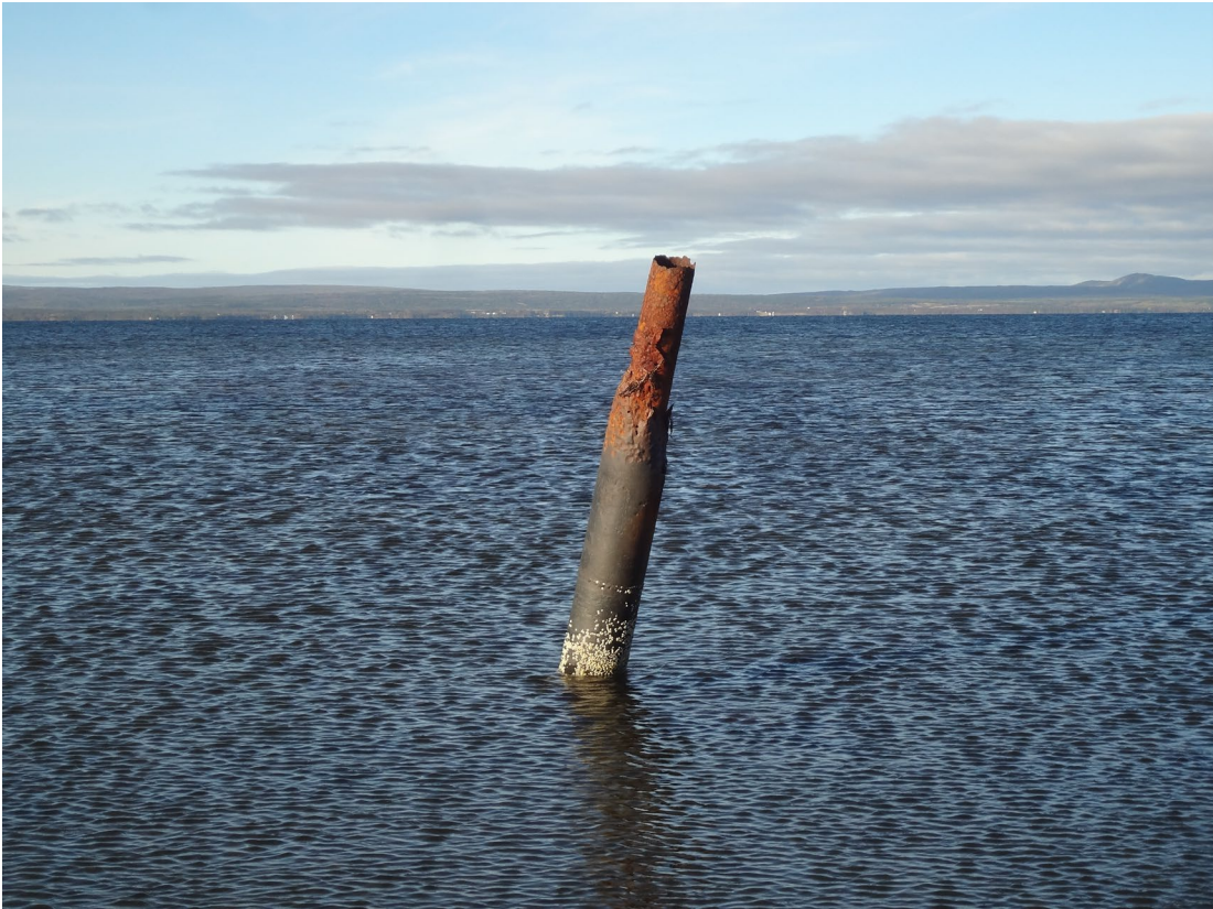
Photo 2 – Abandoned Oil Well Casing (Closest to Shoal Point Tip)
