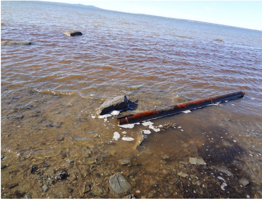
Photo 2 – Location of Well Repair #2
