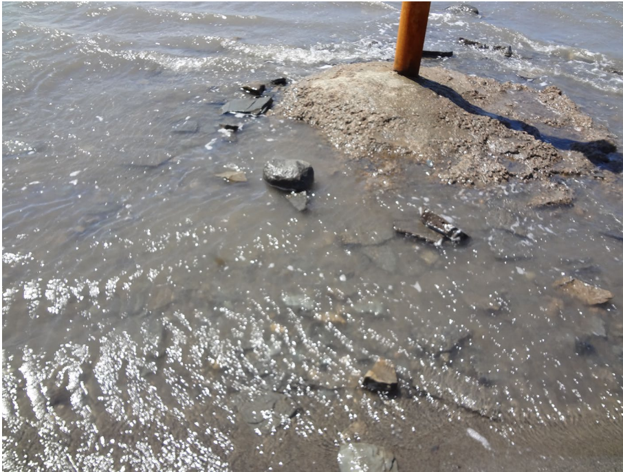
Photo 1 – Concrete base around Well Repair #1
