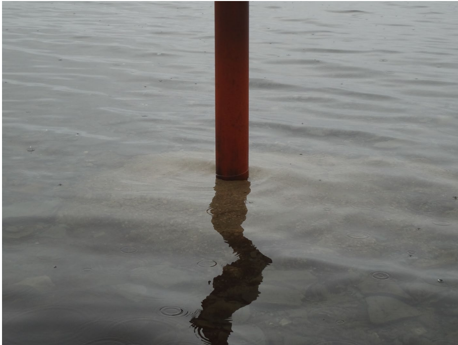
Photo 1 – Base of Well Repair #1
