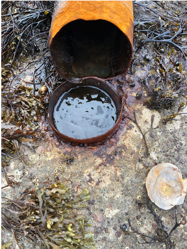
Photo 1 – Pooled Oil/Water Mixture Well Repair #1
