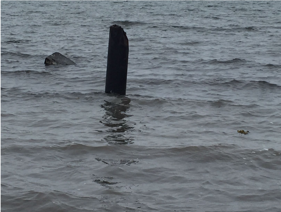
Photo 4 – Abandoned Well Casing
