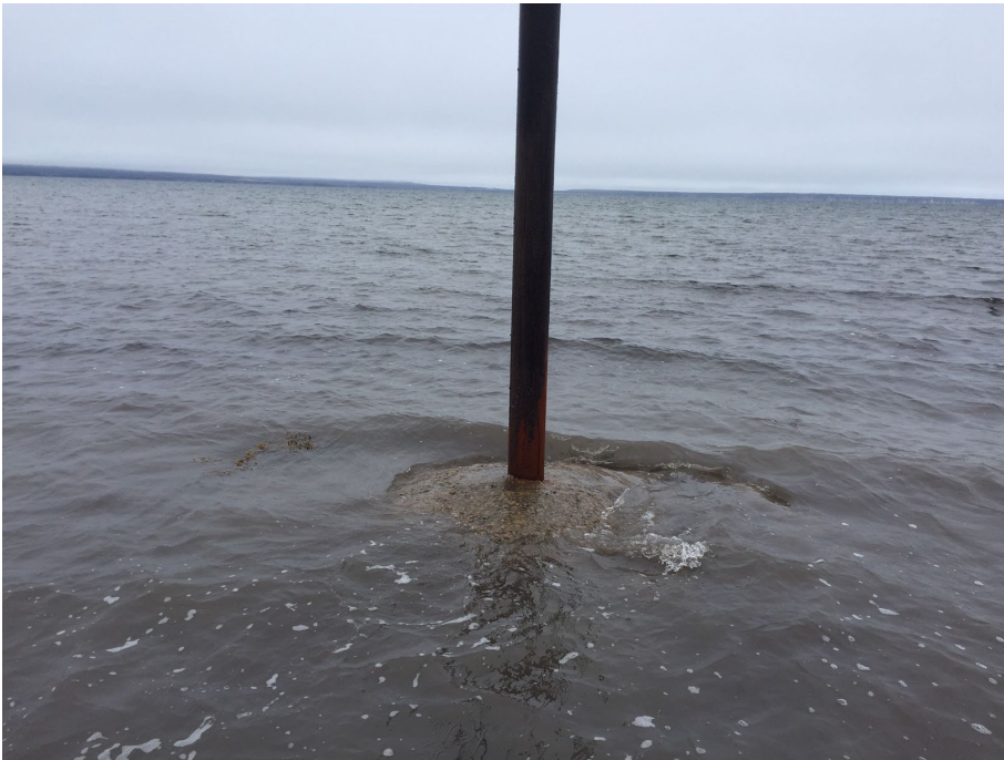
Photo 3 – Well Repair #1 Casing and Concrete Base
