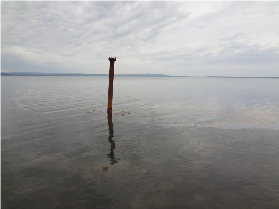
Photo 2 – Oil Sheening in Vicinity of Abandoned Well Repair #1
