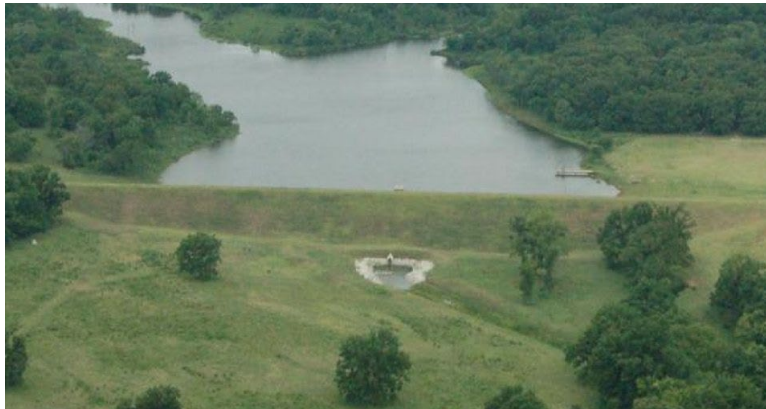
Figure 1: Earthen embankment dam at Double Creek Watershed, Washington County
