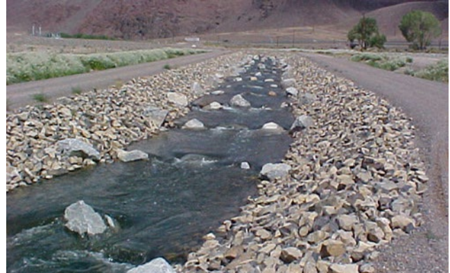
Figure 6: Riprap lined spillway in Truckee River, Nevada
