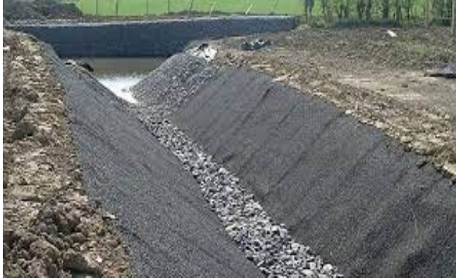
Figure 5: Geotextile lined spillway in Gridley, California
