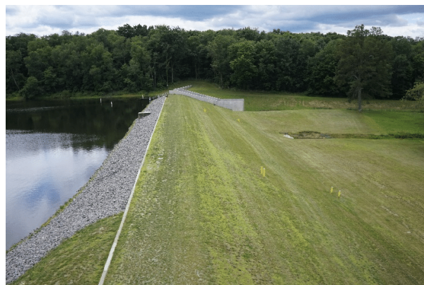
Figure 3: Earthen embankment dam at Glade Run Lake, Pennsylvania
