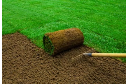
Figure 10: Sod Installation (Sod Installation Costs, n.d.)
