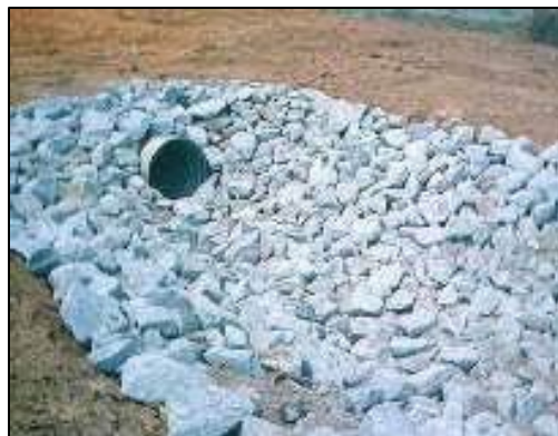
Figure 3: Riprap lined basin
