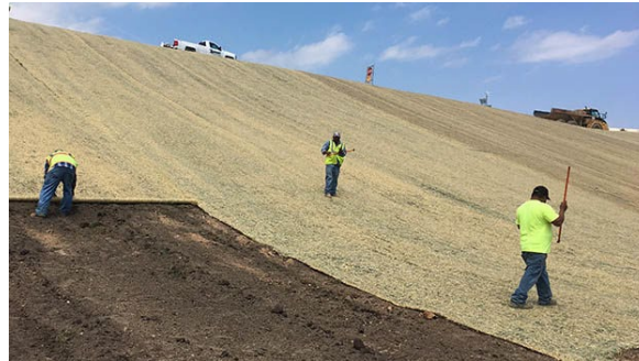
Figure 11: Erosion control blanket (Short Term Erosion Control Blanket, 2021)
