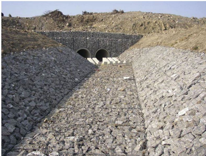
Figure 9: Gabion basket protecting channel against erosion (Channel Lining, 2021)
