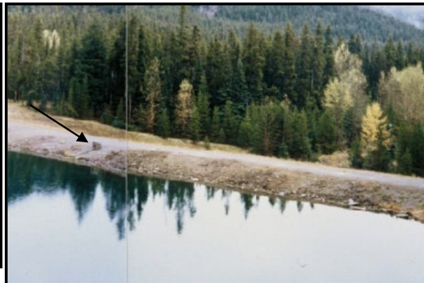
Figure 6: After Remediation: Properly maintained crest and embankment. (FEMA, 2005, Pg. 34).
