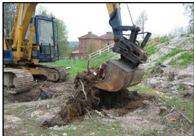
Figure 5 - Stump Pull Test: Removal of Alder stump at Peltokoski embankment dam, Finland. Image retrieved from (Laasonen, 2013, Pg. 2).
