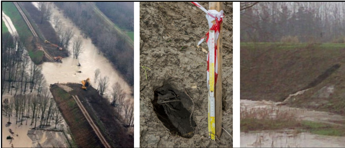
Figure 3 – Left: Significant breach on the Panaro riverbank (Italy) in 2014. The area was known to have significant animal burrows. Middle: Badger footprints and a burrow entrance were observed in 2010 and 2012 at the same area as the breach (left). Right: On the same day as the breach (left), internal erosion caused a smaller breach in an area downstream, which also had animal burrows. Images retrieved from Taccari, 2015, pg. 25 & 134.
