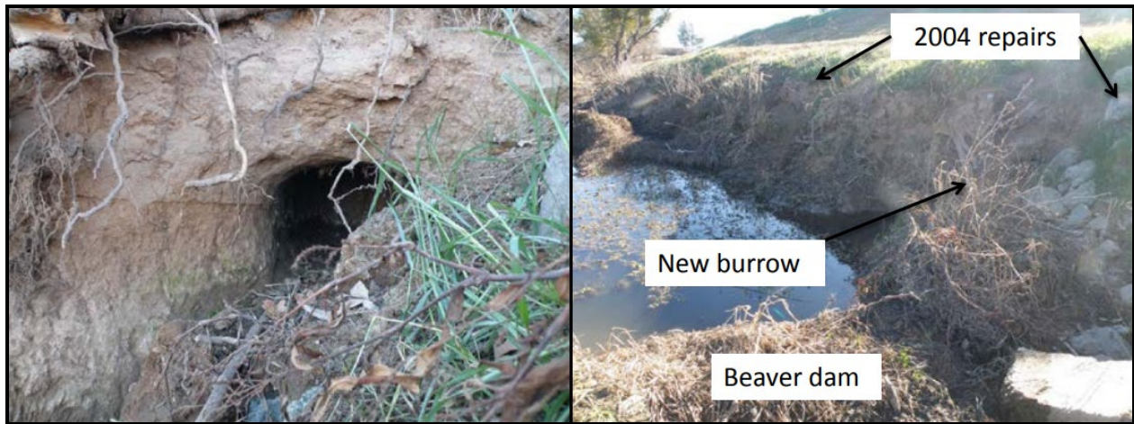
Figure 6 – Left: Entrance to a beaver burrow coincides with tree root (bottom of image), other exposed roots also visible. Right: Reoccurrence of intrusion after a previous repair was completed. Image retrieved from Roa et al, 2014, pg. 41.
